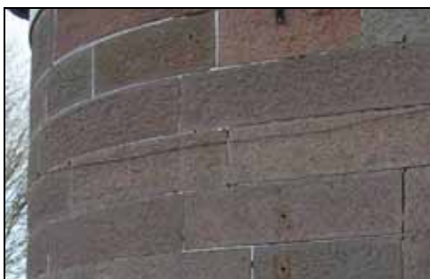
The post office has high quality ashlar jointing and requires repointing soon
