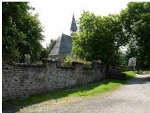
High, Stone retaining wall to the old burial ground
