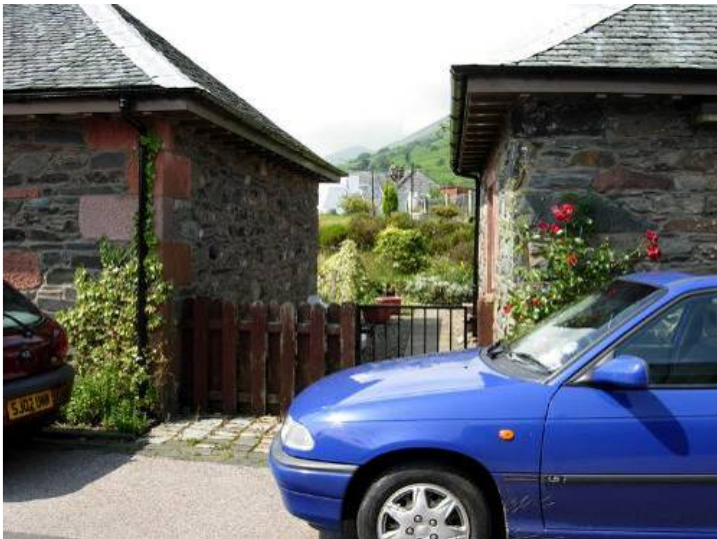
Rubble work and eaves height
