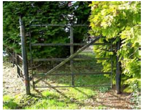
Estate railings to the cemetery
