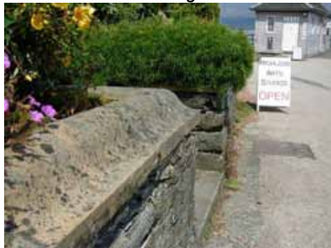
Fine stone copings to the front of Lochview & Pierhead
