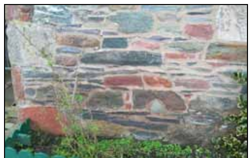
Flower beds adjacent to walls encourage soaking of the wall base, in some cases this is leading to washing out of the mortar NB the mortar mix here is questionable
