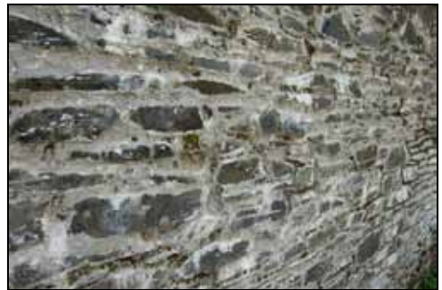
Church wall, recently pointed but the mix is questionable and is deteriorating rapidly
