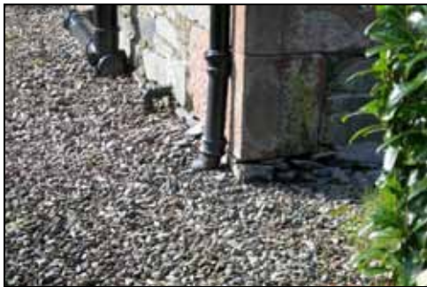
Poorly detailed rainwater disposal leading to washing out of mortar from base of wall – Dell Cottage
