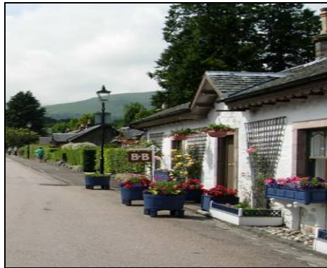
Tigh a Mhaioir with decorative fascias and vertical sash windows
