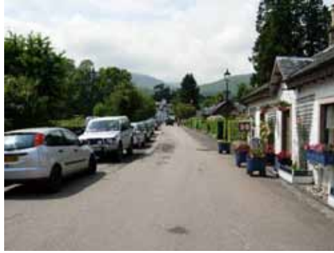
The western extension of the main street, the view terminated by the Colquhoun Arms Hotel.
