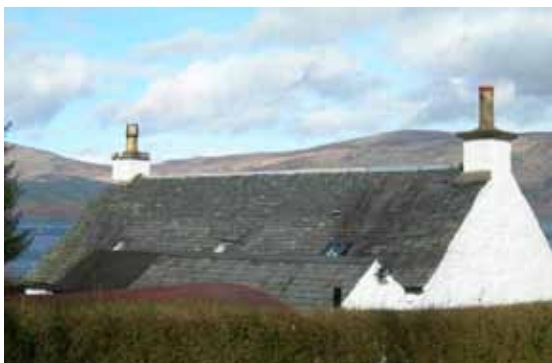
Rear view of Shore Cottage
