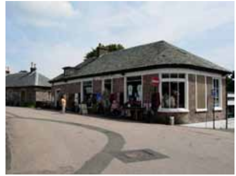
The Post Office junction of main street, School Road and curving lane
