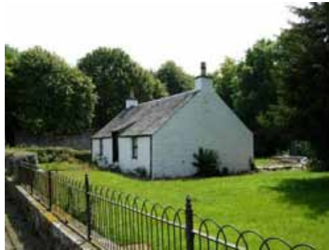
Wrought iron railings on the Shore
