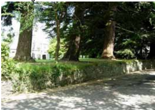
Retaining wall to the cemetery
