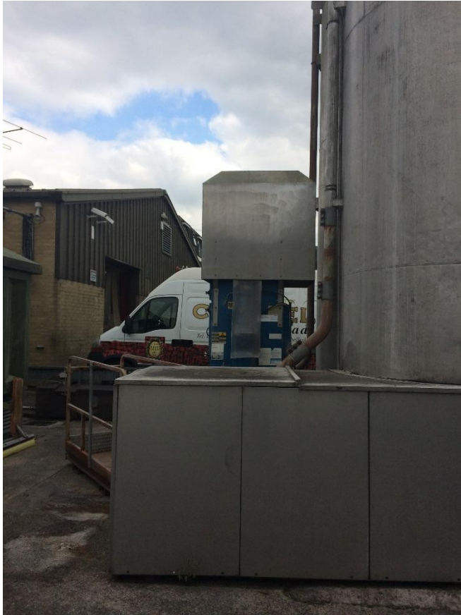
Edge of Silos and warehouse building
