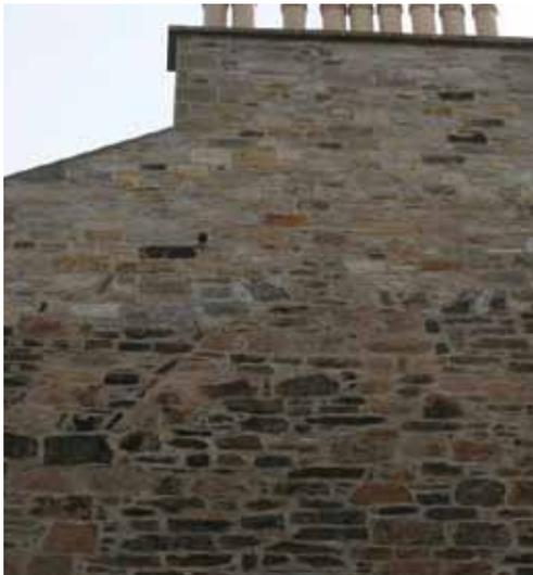
*Fig. 2 Diagonal bridges made from stone slabs, visible on the gable end of this tenement in Edinburgh, indicate the presence of flues within the wall.*
