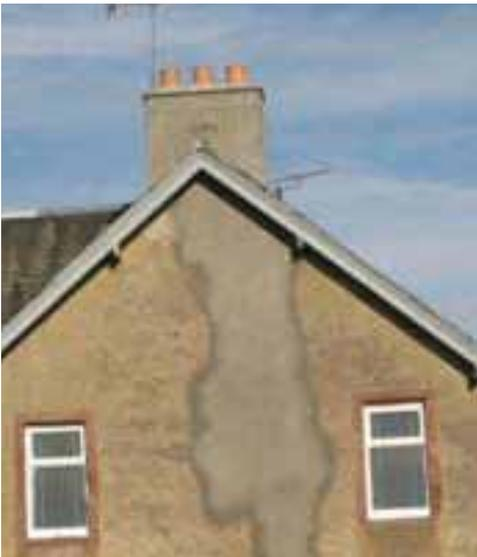
**Fig. 9** A flue relined from the outside.
