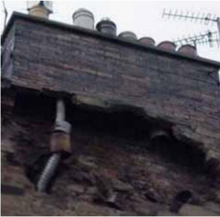
**Fig. 8** Collapse of parts of a gable due to washed out mortar.
