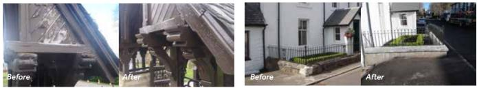
This work was carried out by skilled masons using a traditional lime mix which matched the original mortar. The work also revealed that the building was originally longer than it is now extending out into an area now occupied by the lane.
