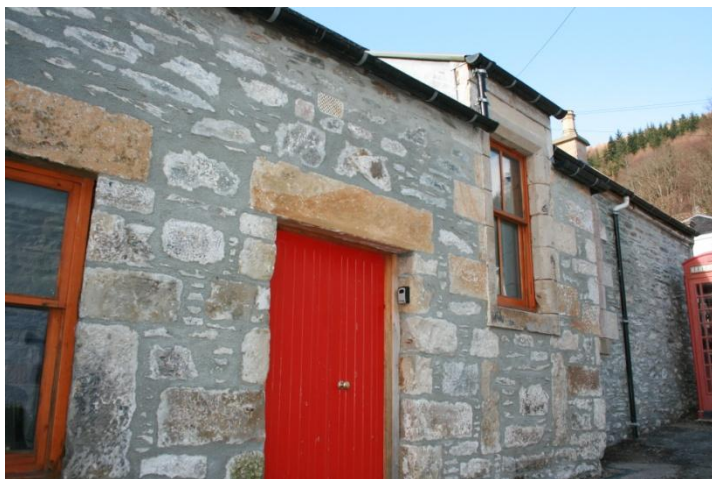
1. Kilmun Pier - re-pointing of listed former Post Office House
