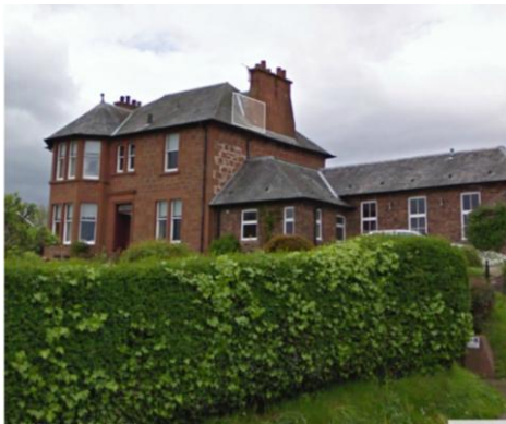
Ashbank, Drymen – sash and case window refurbishment.
