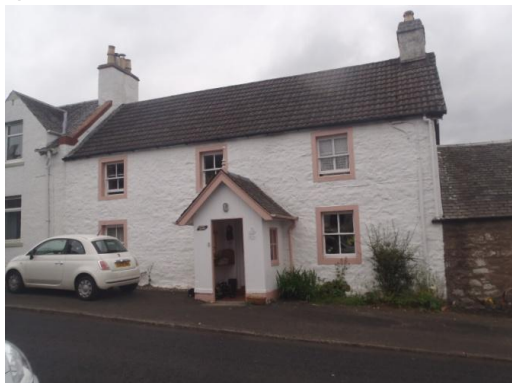
Murray House , Gartmore – replacing concrete roof tiles with slate.
