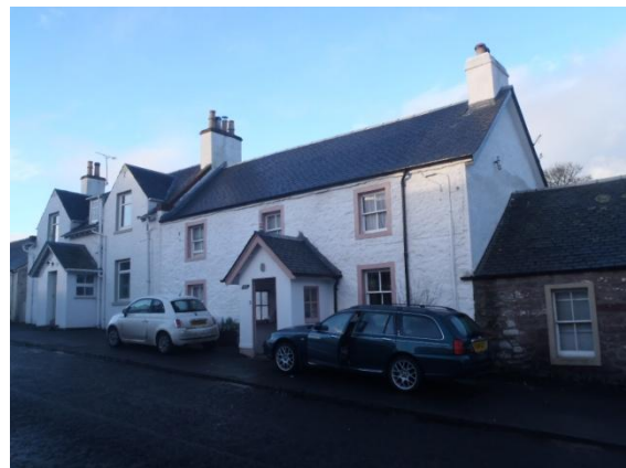
Murray House, Gartmore – replacement of concrete tiled roof with slate.
