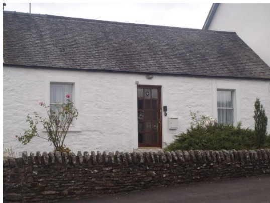
Hazel Cottage, Gartmore – replacement of non-traditional windows and door, with timber sash and case double glazed units and traditional style timber door with matching glazing pattern.
