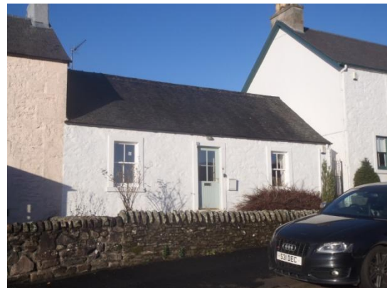
Hazel Cottage, Gartmore – replacement of non-traditional windows and door, with timber sash and case double glazed units and traditional style timber door with matching glazing pattern.
