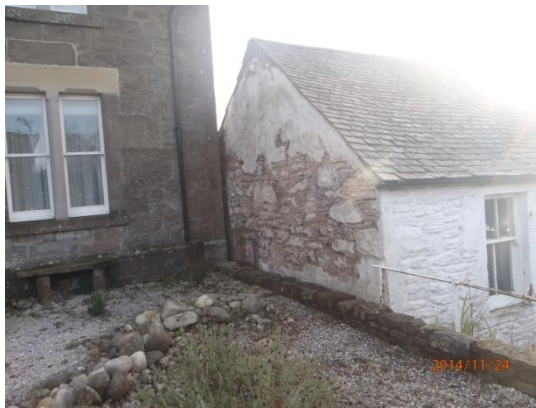
Cobblers Cottage, Gartmore – removal of paint and re-pointing with lime mortar
