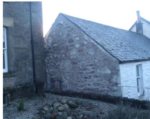
Cobblers Cottage, Gartmore – removal of paint and re-pointing with lime mortar
