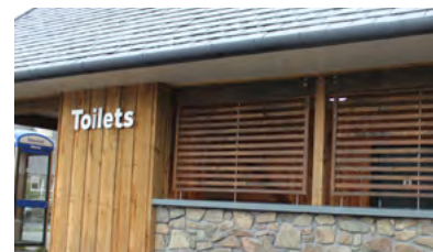
Stone and wood cladding
