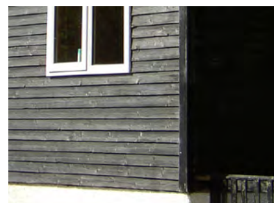
Glenbranter, Timber cladding
