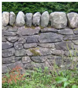
The Glassert, Boundary wall
