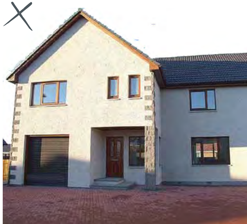
Poor choice of materials; heavy roof tiles; visually intrusive construction detail at eaves and verge; cast stone quoins; poor fenestration
