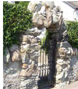
Strone, Rubble wall and arch
