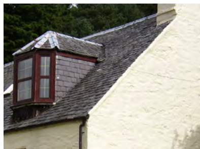
Loch Eck, painted rubble walls, slate roof
