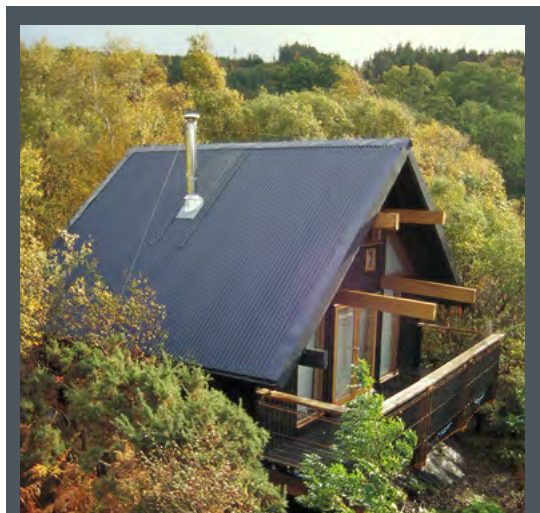
This timber house near Oban incorporates a system for the collection and use of rainwater as the sole source of domestic water and has a reed-bed filtration system which treats sewerage.
