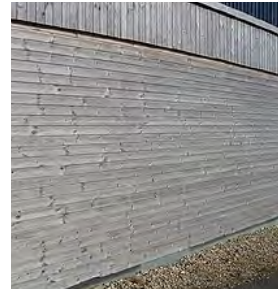
Weathered larch cladding
