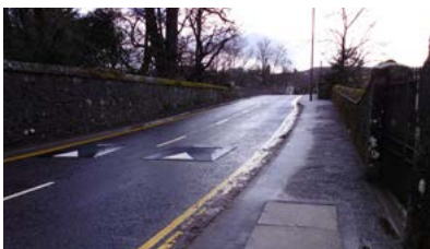
Road bridge along A81 is listed and is only capable of pedestrian access on western side of road
