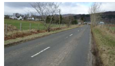
A81 potential roundabout access point to Claish Farm and gateway approach from south
