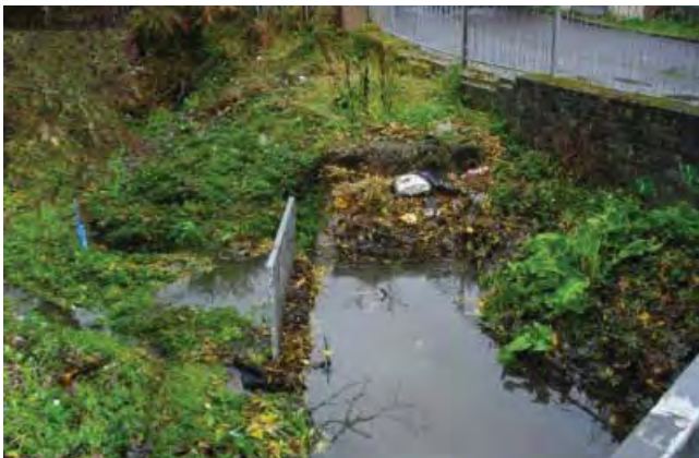
Blocked culvert
