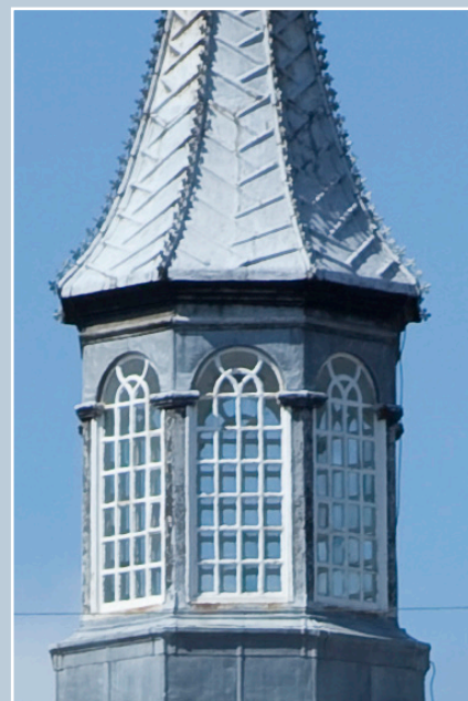
Fixed small-pane windows in the cupola of Robert Gordon's Hospital, Aberdeen, designed by William Adam in 1731–32. Thick astragals (glazing bars) and small panes of glass are typical of this period of design. © N. Haynes.
