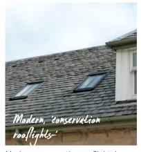
Modern conservation rooflight, low profile, metal, top hung with vertical glazing bar reflecting traditional features.
