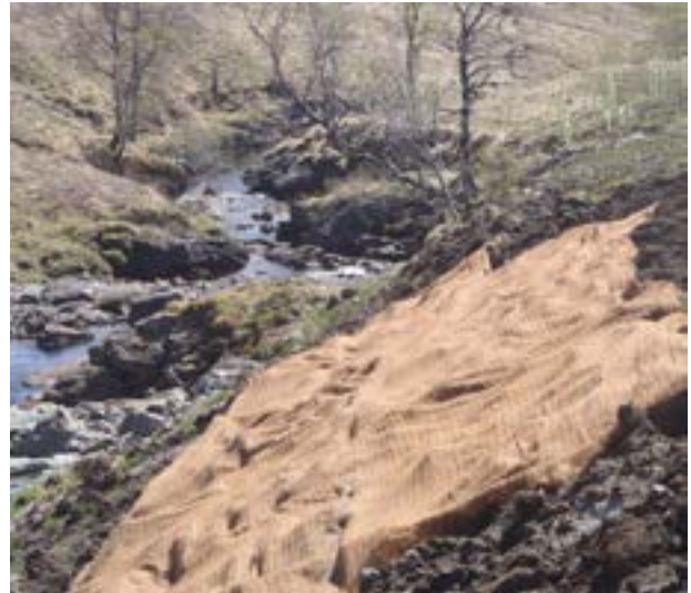
Figure 12: Use of Geo-textile to stabilise and help colonise bank.
