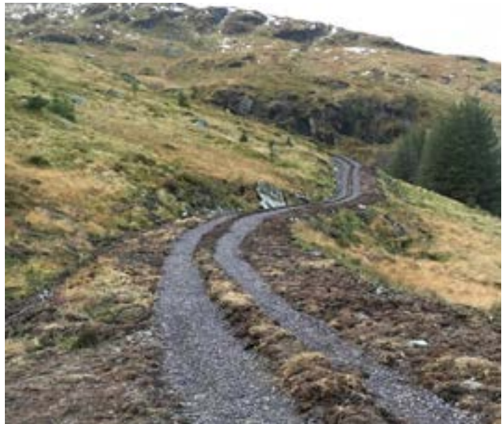
Figure 4 Track reduced in width post construction and strip created in centre added to speed up restoration
