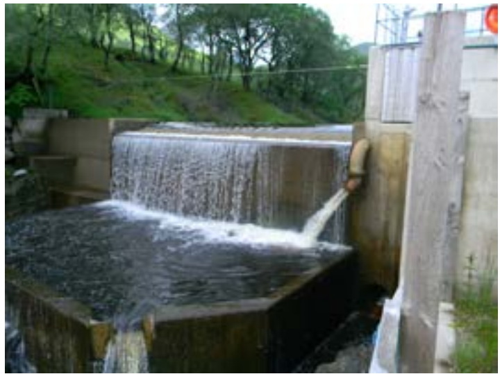
Figure 10 Intake showing concrete coloured by water flow
