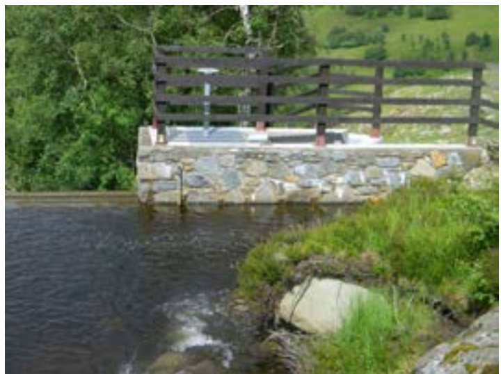
Figure 11 Wing walls with stone facing
