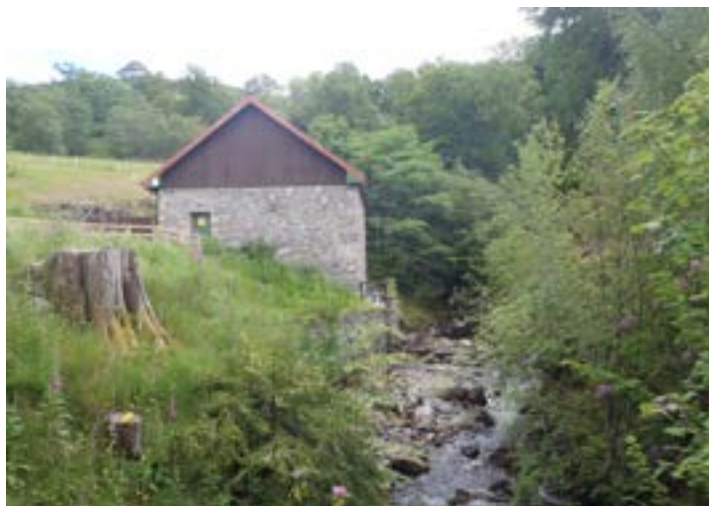
Figure 7: Powerhouse making use of former mill ruins
