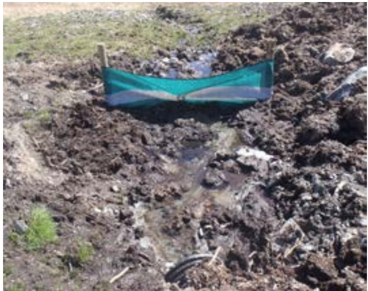
Figure 2: Silt trap below culvert
