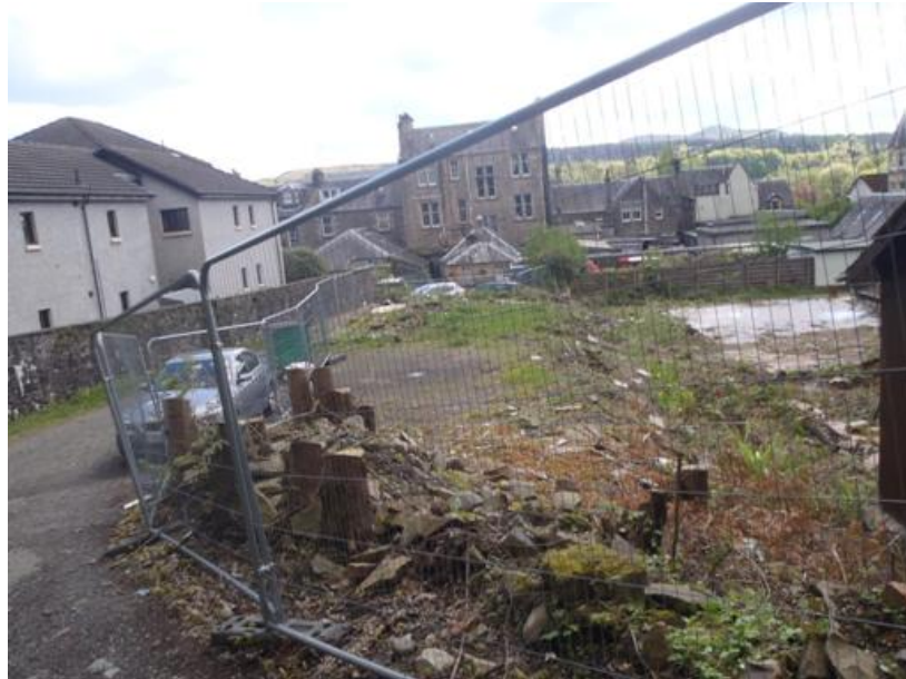
View of Site from Existing Rear Access Lane
