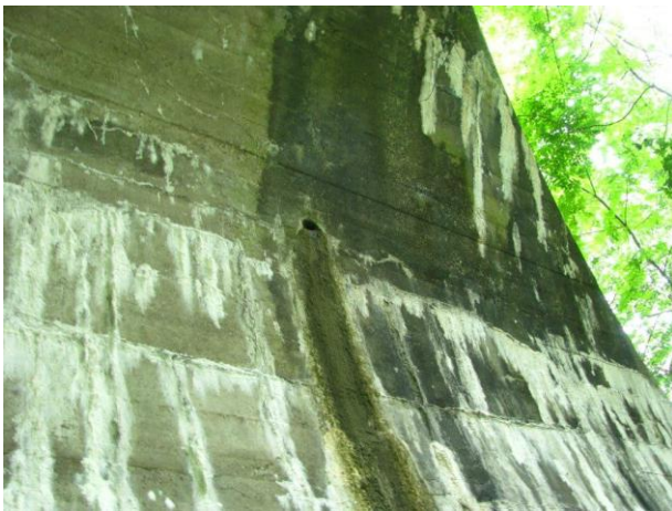
Fig. 6: Existing drainage hole
