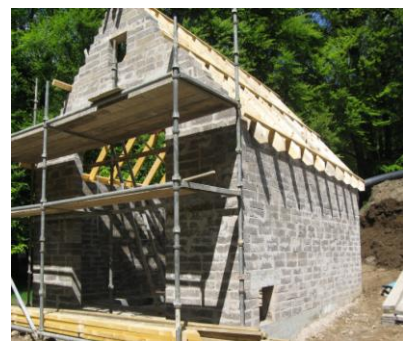
Stronchullin Hydro Scheme Powerhouse
