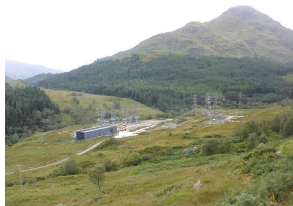
Sloy Electricity Switching Station Before and After Removal of external switching station and building and replacement with single contained building
