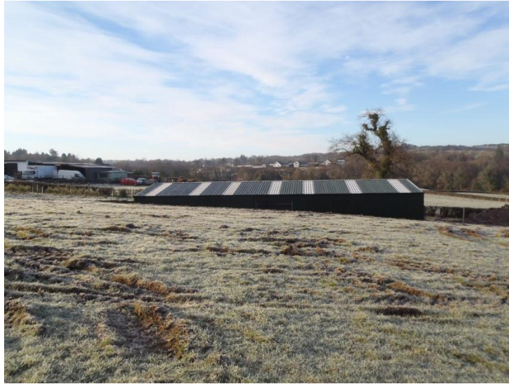
Fig.3. View to shed from north east illustrating ground profile. France Farm in background.
