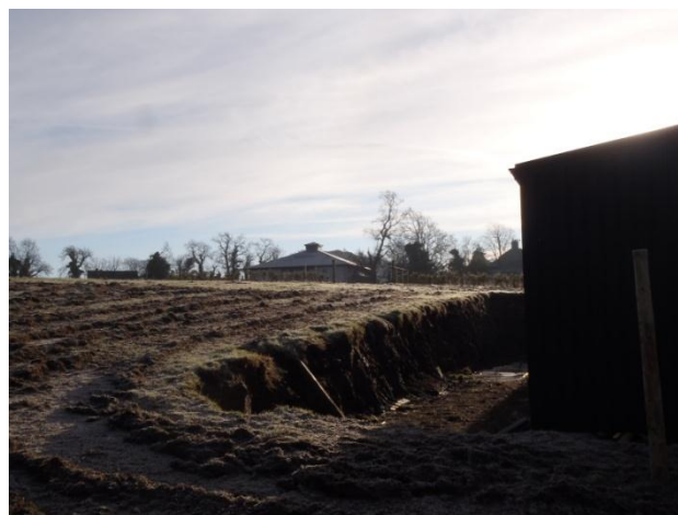
Fig.5. View from shed showing excavated banking, the field and Millennium Hall.
