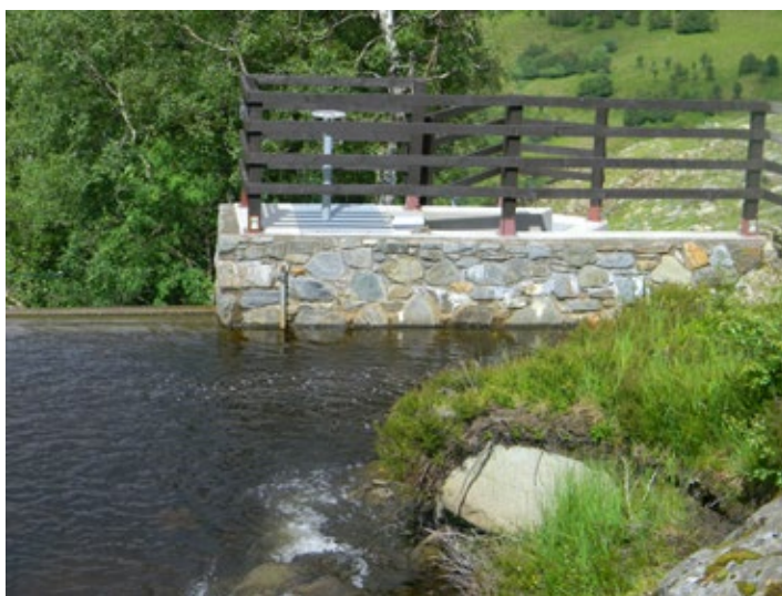
Figure 11 Wing walls with stone facing
