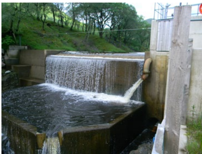
Figure 10 Intake showing concrete coloured by water flow
