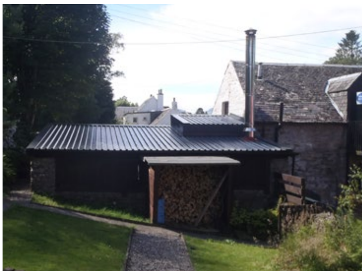
Figure 17: Biomass facility in outbuilding
