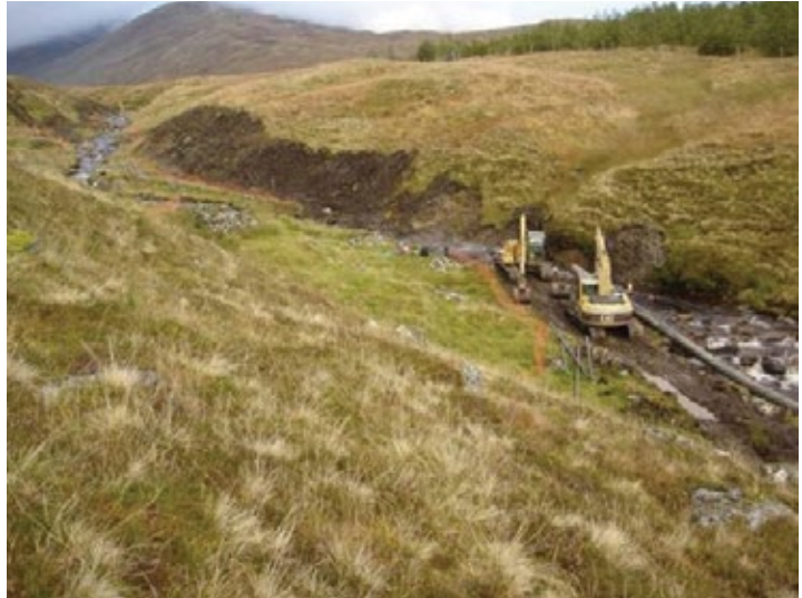
Figure 8: Penstock Route: note working corridor is limited and exclusion area marked on ground with temporary fencing
