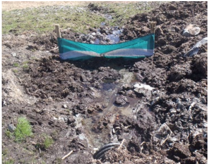
Figure 2: Silt trap below culvert
