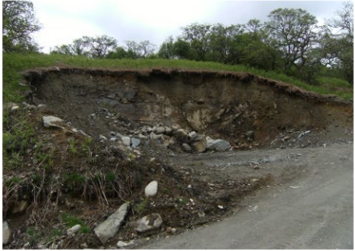
Figure 6: Borrow pit prior to restoration
