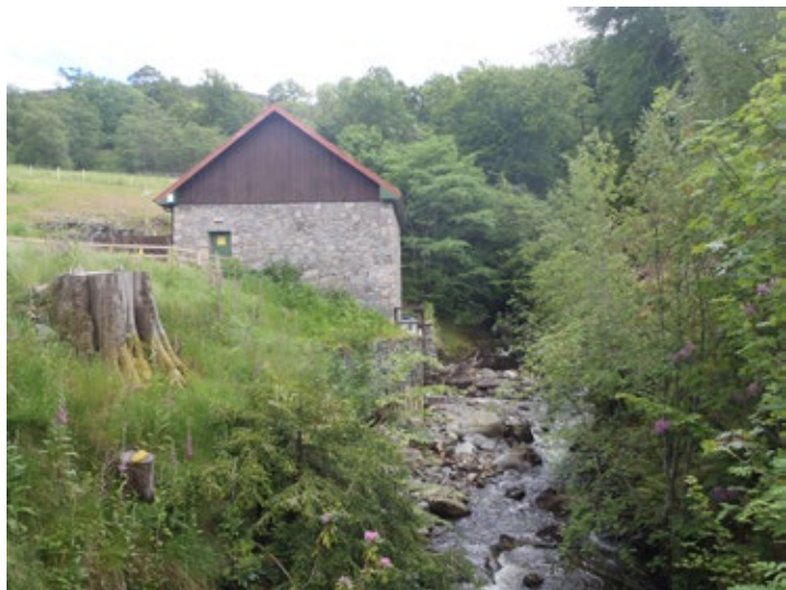
Figure 7: Powerhouse making use of former mill ruins
