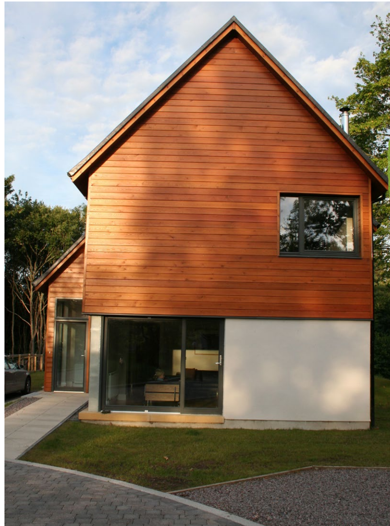
Treated timber cladding
