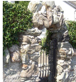
Strone, Rubble wall and arch
