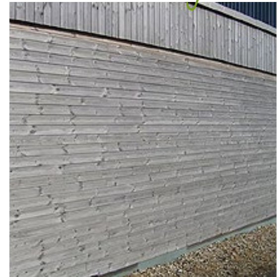
Weathered larch cladding
