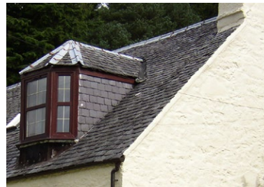
Loch Eck, painted rubble walls, slate roof
