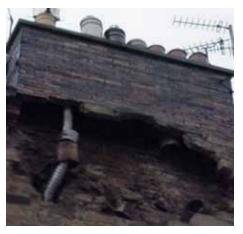
Fig. 8 Collapse of parts of a gable due to washed out mortar.
