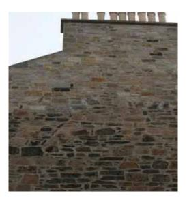
Fig. 2 Diagonal bridges made from stone slabs, visible on the gable end of this tenement in Edinburgh, indicate the presence of flues within the wall.
