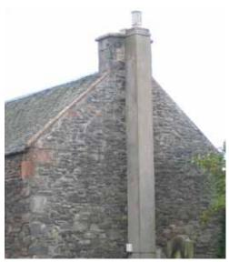
Fig. 10 A new flue built onto the exterior face of a gable.
