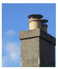
Fig. 7 Conical cover for a chimney can.
