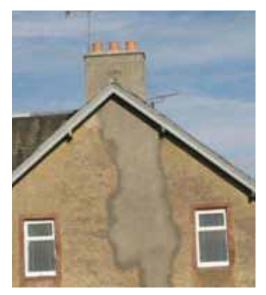
Fig. 9 A flue relined from the outside.
