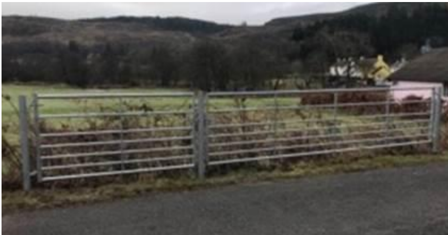
Photograph 12: New field gate (permitted development)
