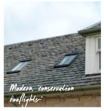
Modern conservation rooflight, low profile, metal, top hung with vertical glazing bar reflecting traditional features.
