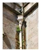
Faulty rainwater goods can result in vegetation growth and staining and damage to stonework.
