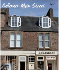
Good example of matching pair of dormers with sliding timber sash and case double glazing
