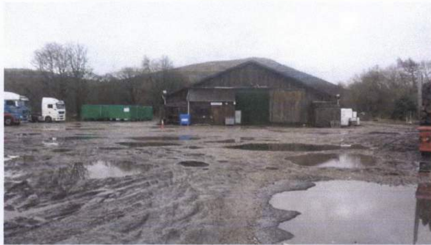
Plate 16 – Looking northeast towards the sawmill buildings across the transport staging area.
