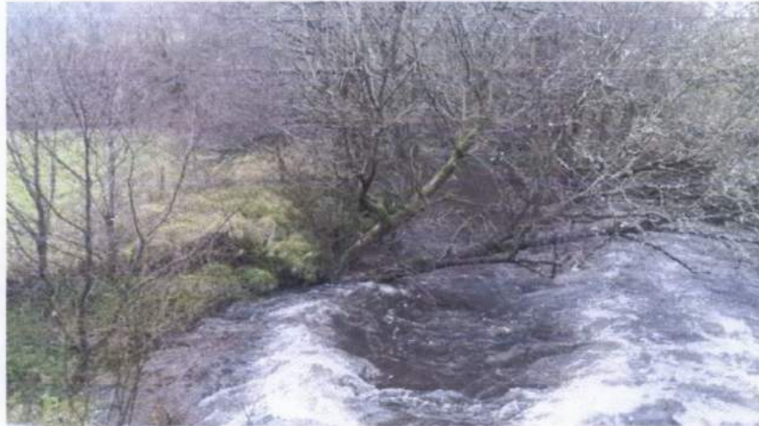
Plate 13 – View west from A815 Road Bridge of the River Cur (downstream).
