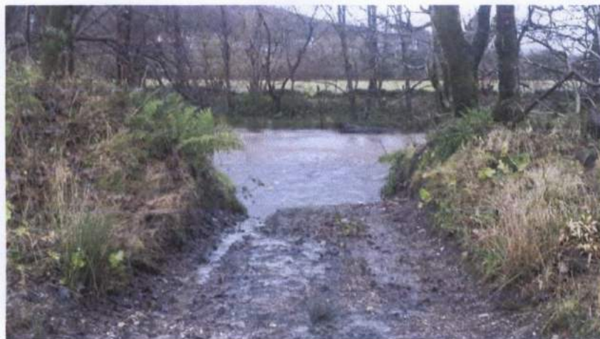
Plate 18 – River Cur embankment cut through, upstream of the site.
