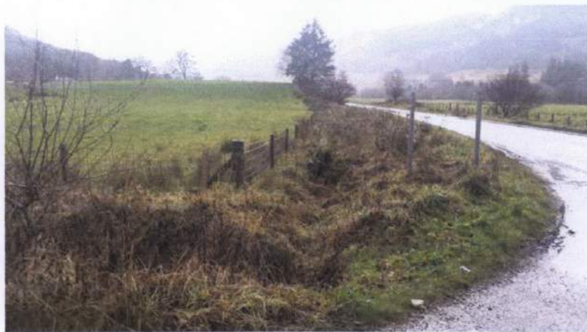
Plate 3 – View south showing drainage ditches around the site access.
