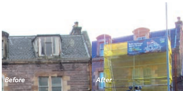
Main St, Callander Reinstatement of Traditional Stone Dormer
