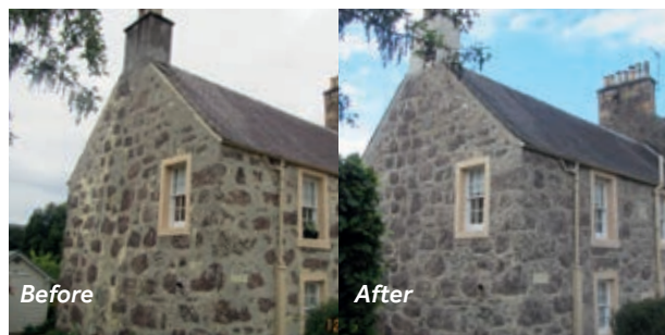
Callander Repointing with Traditional Lime Mortar
