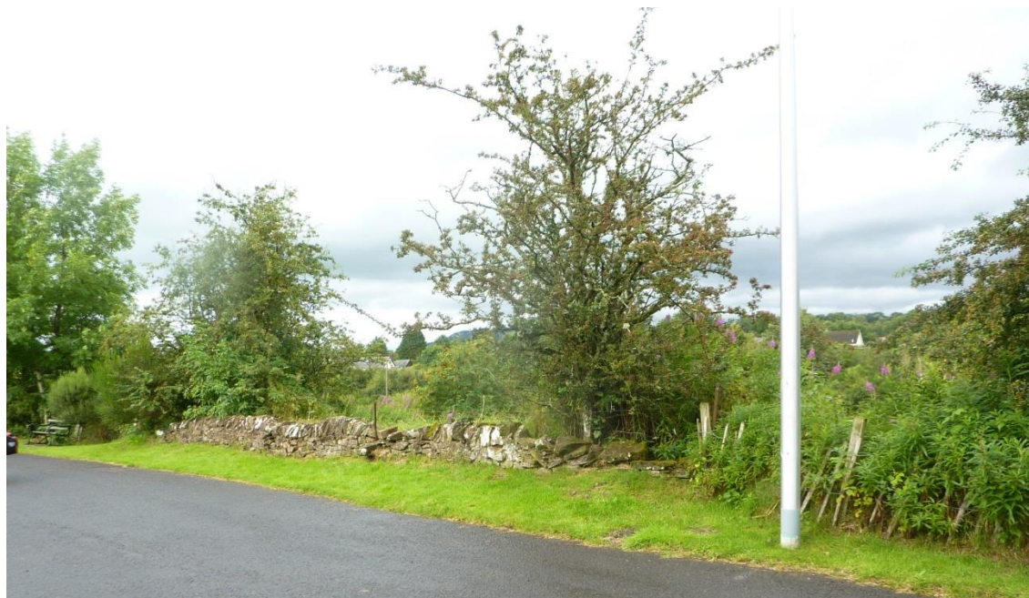
Figure 15: Drystone Dyke on Gartness Road; proposed to be retained and repaired.
