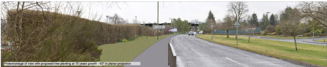
Figure 19c: View of the site from the A81 looking south (in Year 15)
