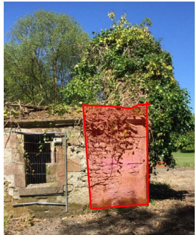
Photograph 21 – East end of South elevation of south block Showing bulging wall and down takings in red
