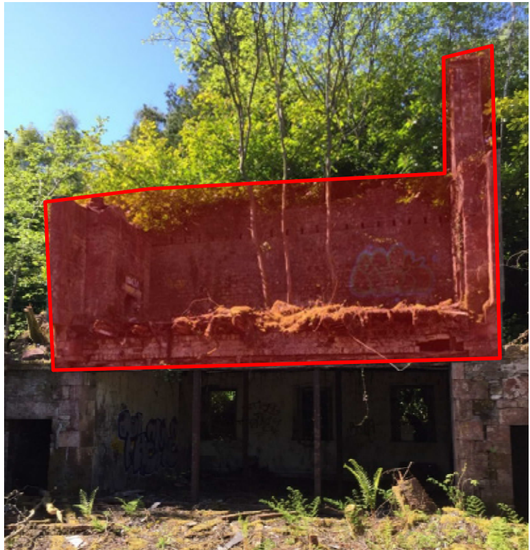
Photograph 24 – first floor of rear section Showing priority down takings for safety in red
