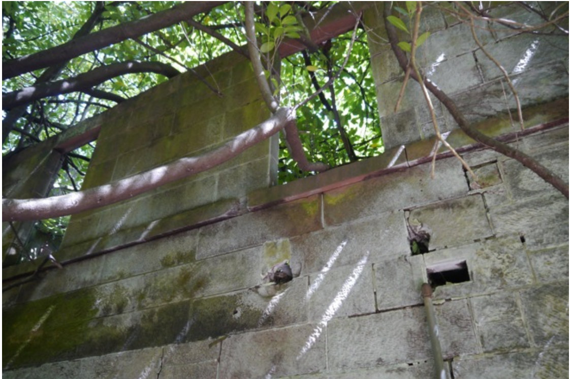
Rear of rear section - overwhelmed by tree growth - now causing structural damage.
