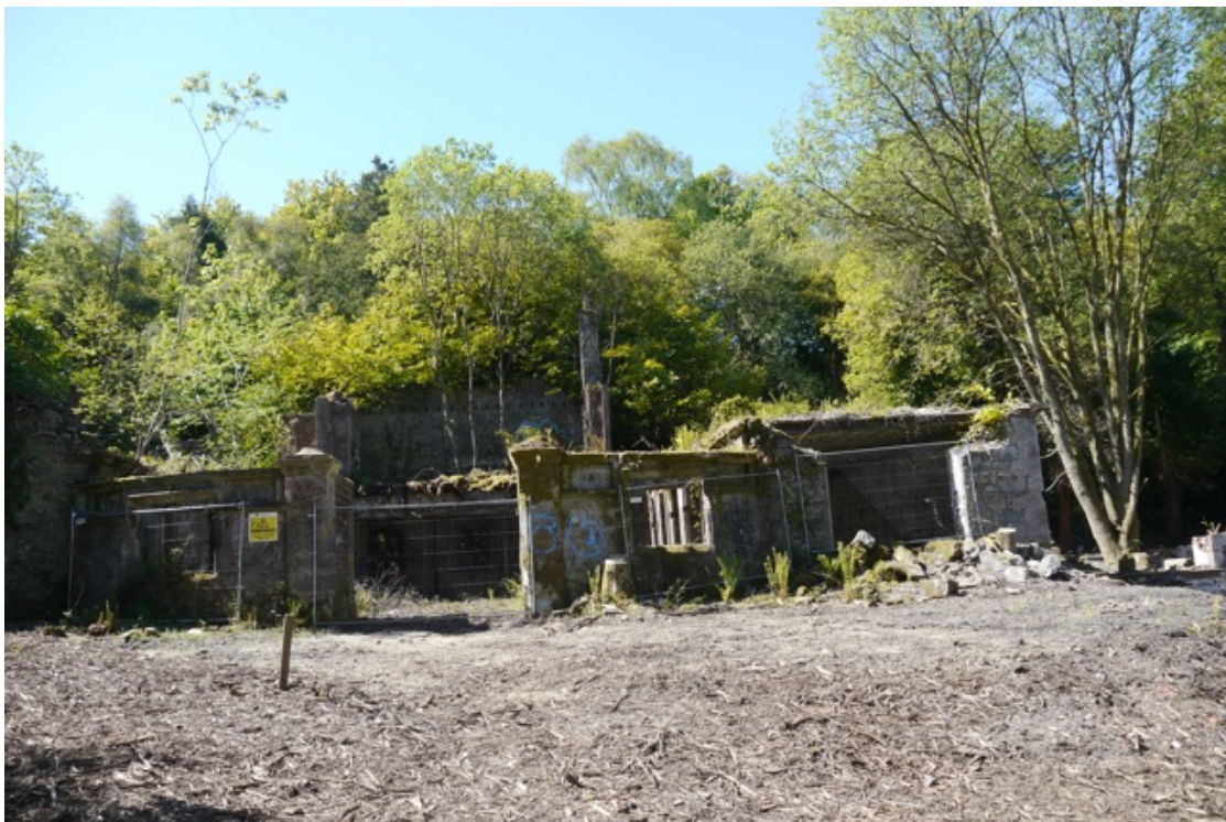
Central entrance with curved wall to courtyard and collapsed gable to north block.
