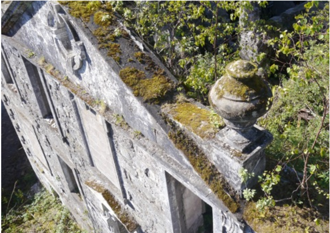
Above and below - pediment stonework is relatively sound.
