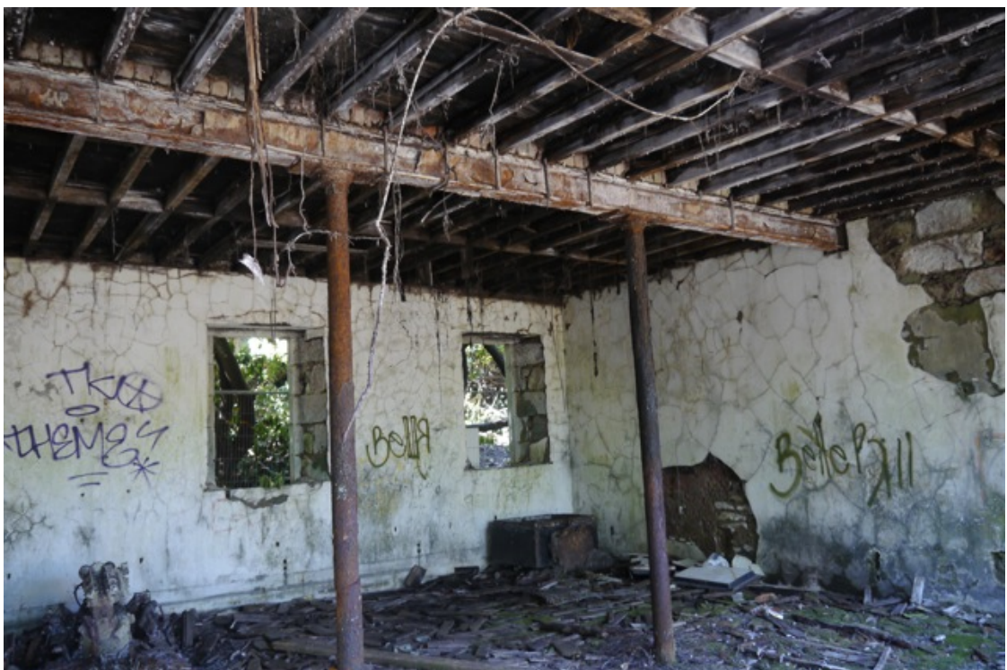
2-storey rear section: above - note mature trees growing out of first floor structure; below - note shear crack in left-hand column (supporting brick spine wall).
