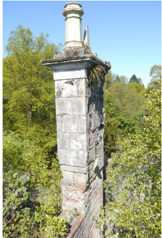
Above - structurally unstable central chimneys and vegetation growing off concrete second floor.
