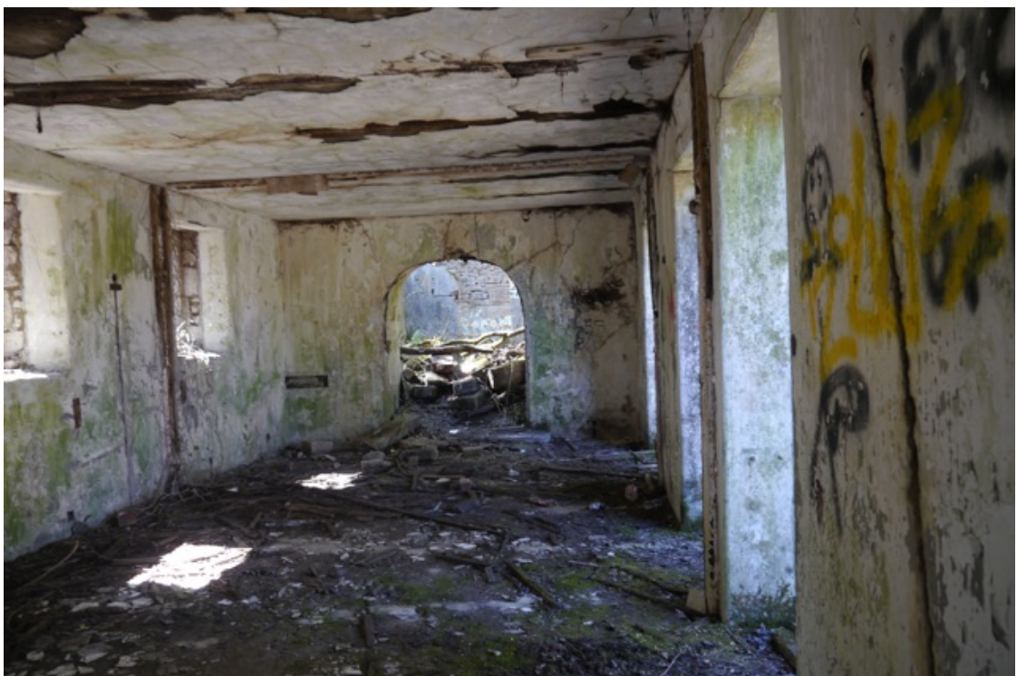
Below - within south block - ceiling still intact despite collapsed roof.
