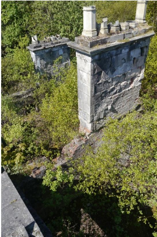
Above - structurally unstable central chimneys and vegetation growing off concrete second floor.
