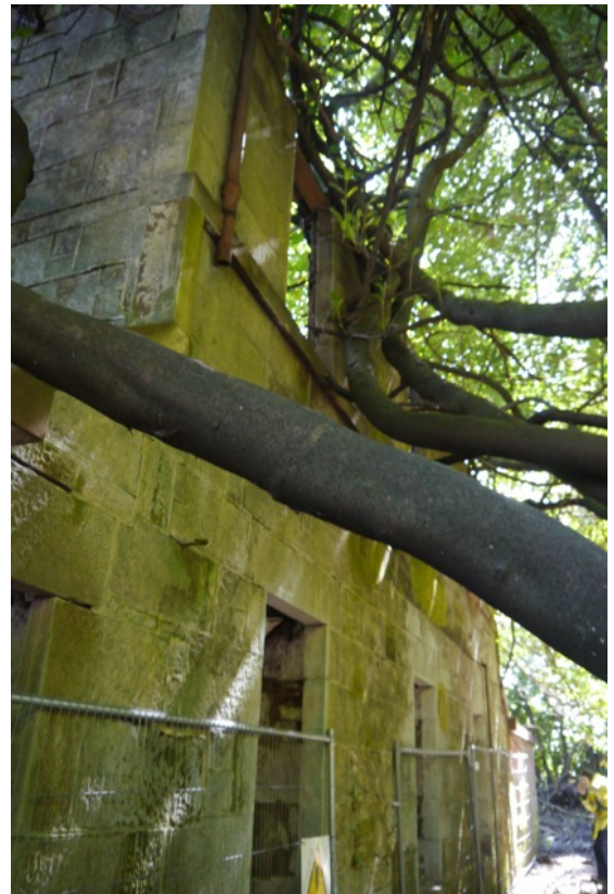
Rear of rear section - overwhelmed by tree growth - now causing structural damage.
