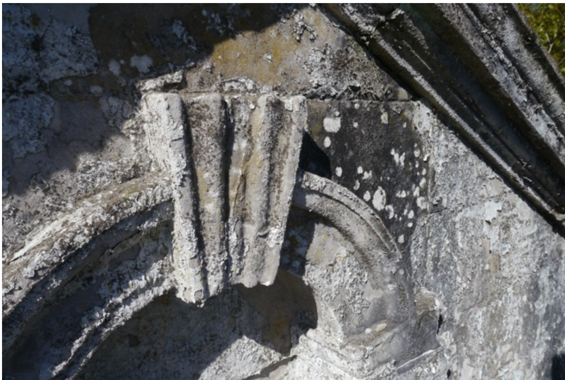
Lichen and flaking masonry paint on stone pediment.
