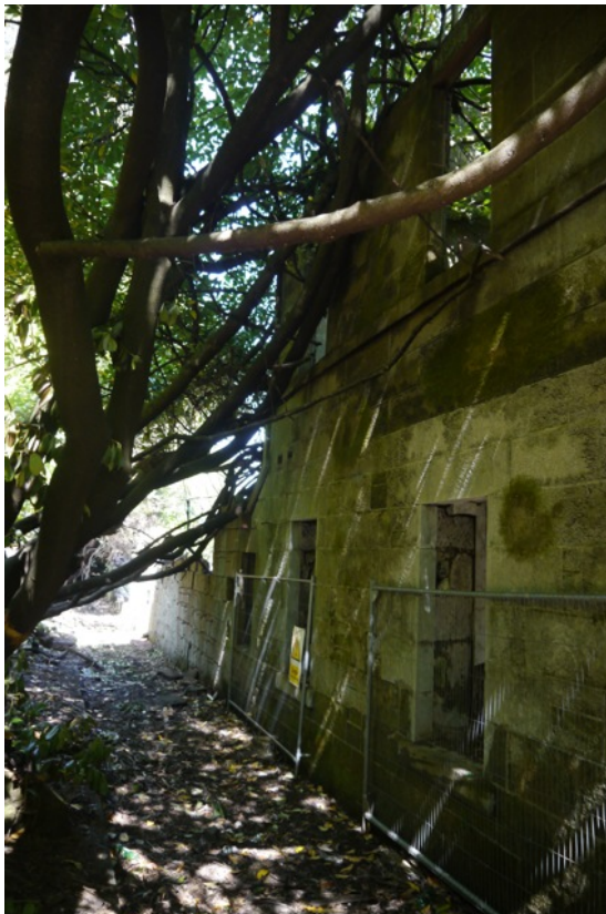
Rear of rear section - overwhelmed by tree growth - now causing structural damage.
