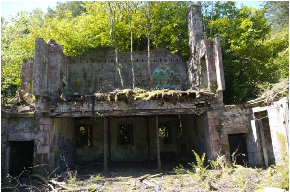
2-storey rear section: above - note mature trees growing out of first floor structure; below - note shear crack in left-hand column (supporting brick spine wall).
