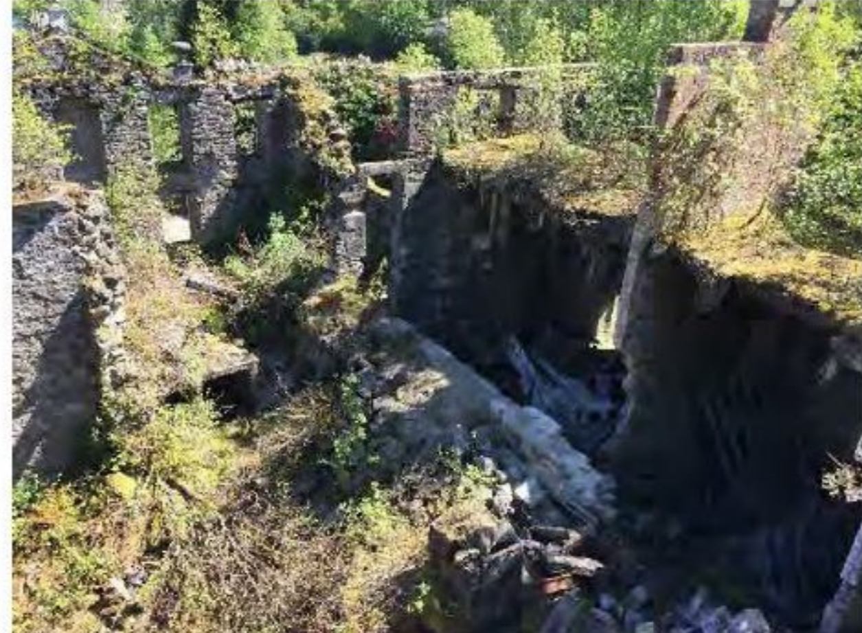
Photograph 16 - Internals from South west
