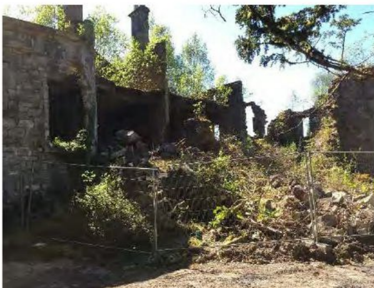
Photograph 15 - Internals from North
