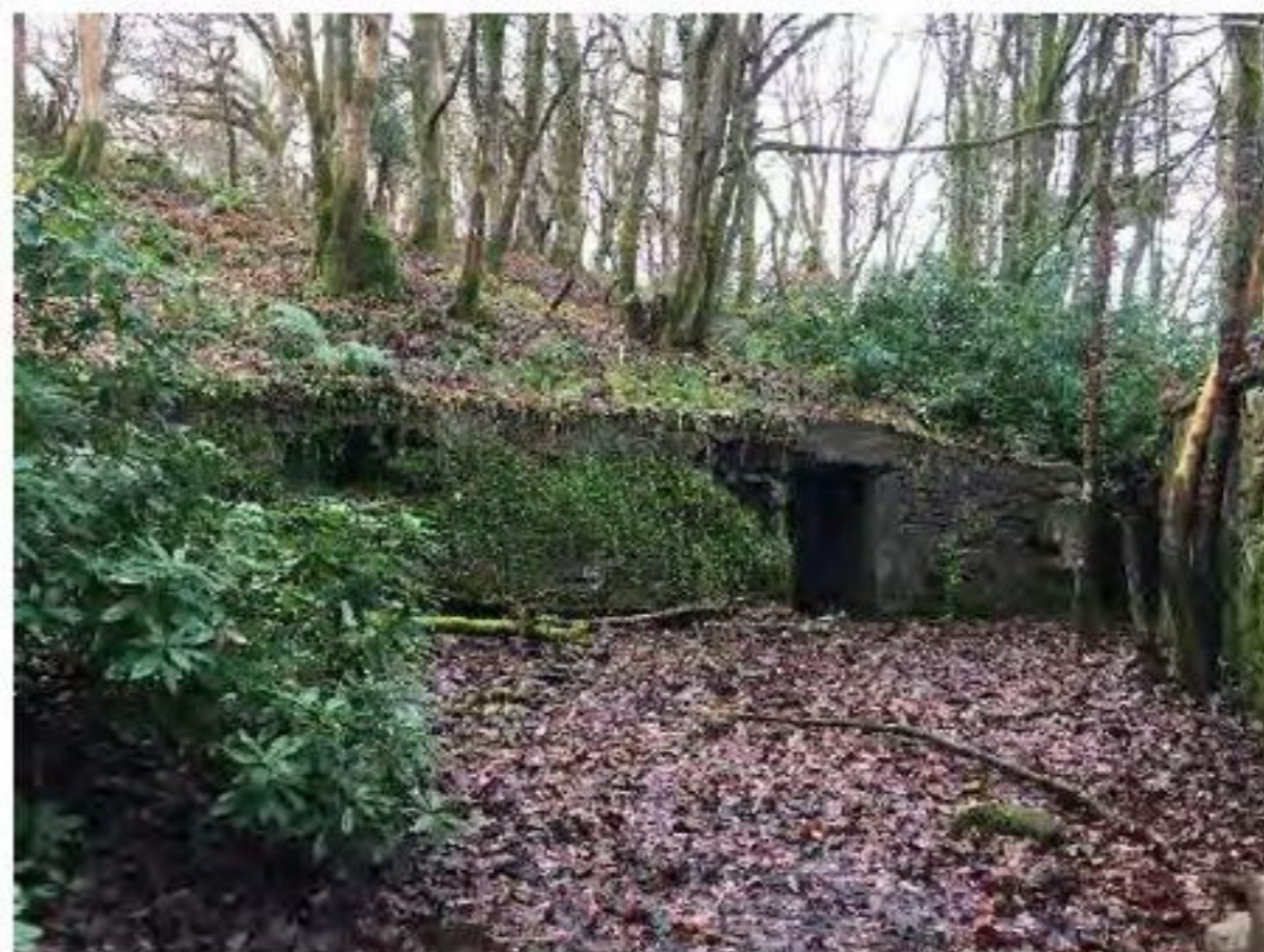
Photograph 33 – South West Retaining wall
