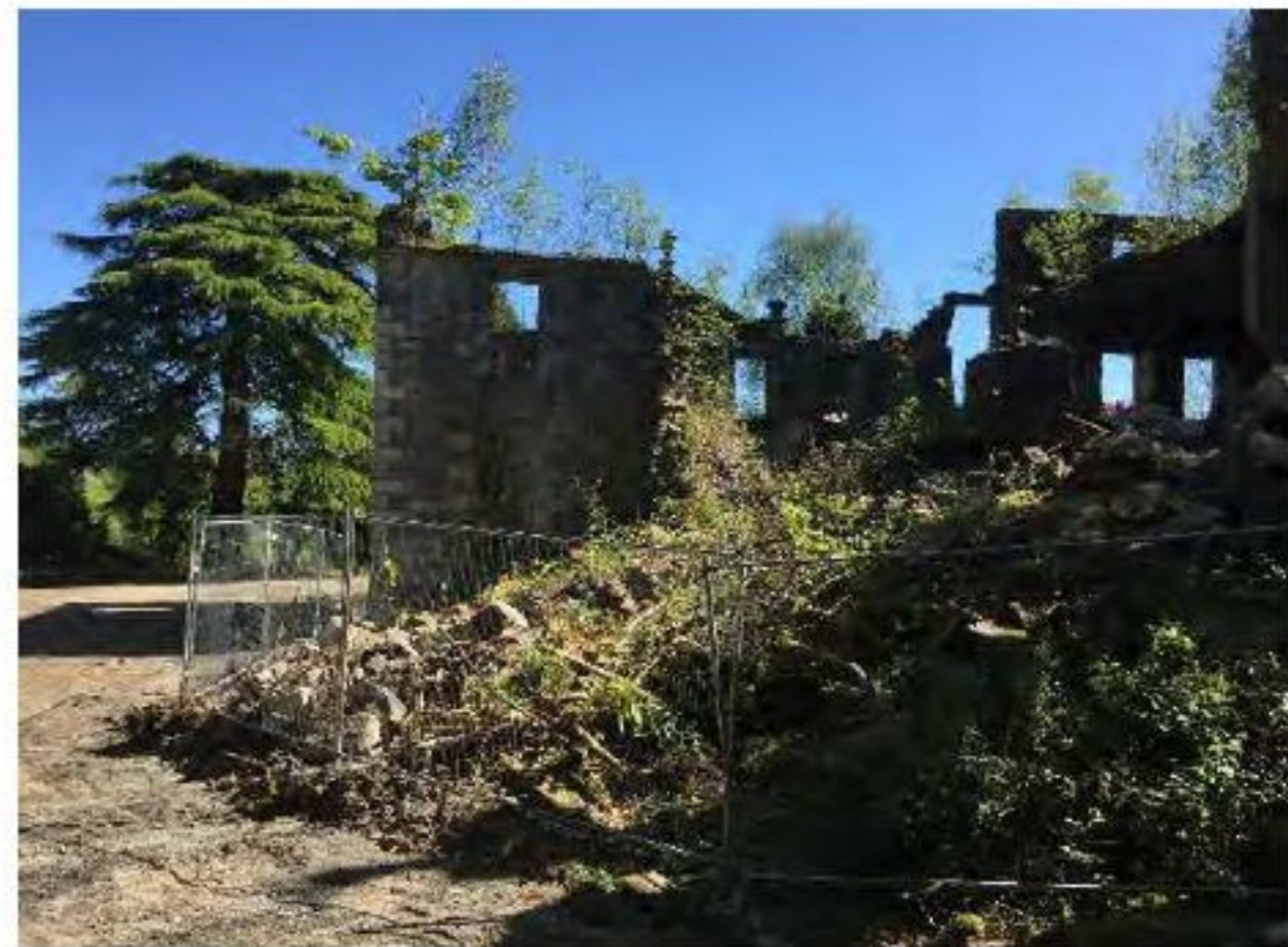
Photograph 14 - Internals from South
