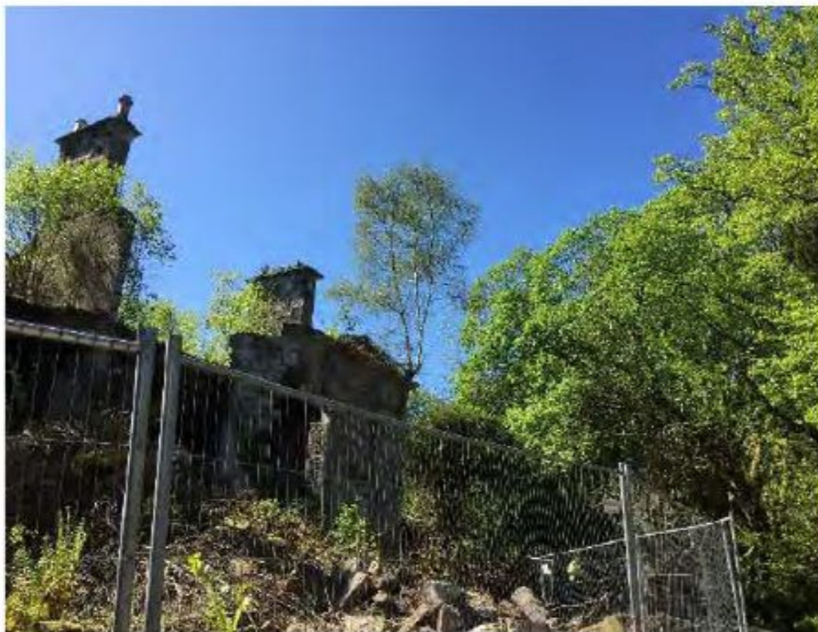
Photograph 13 - Internals from North east
