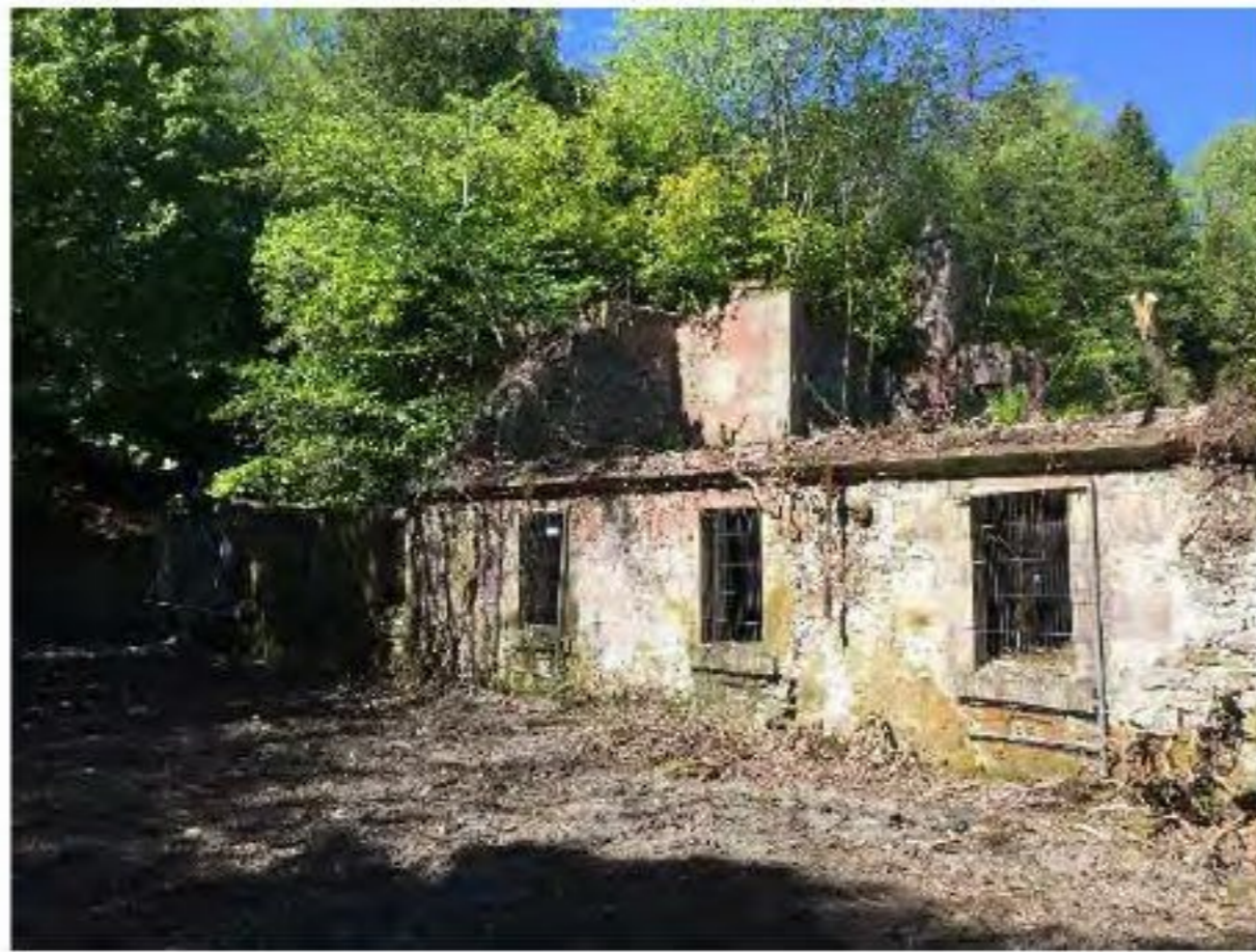
Photograph 19 – South elevation of south block
