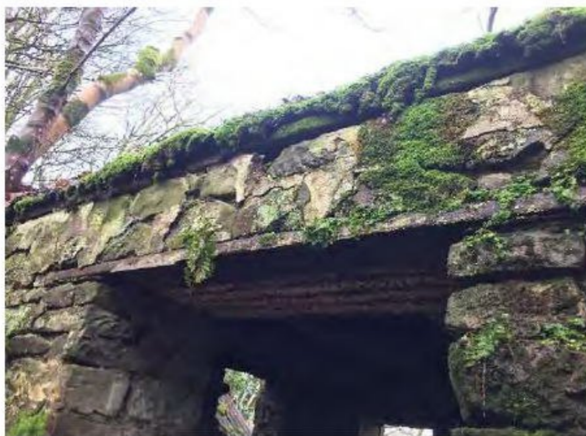
Photograph 31 – West wall lintel, formed with rails
