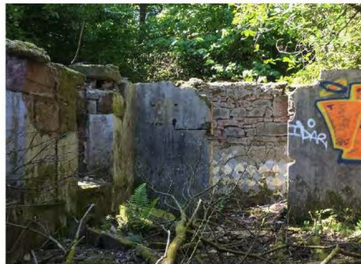
Photograph 18 – Internal views of south block
