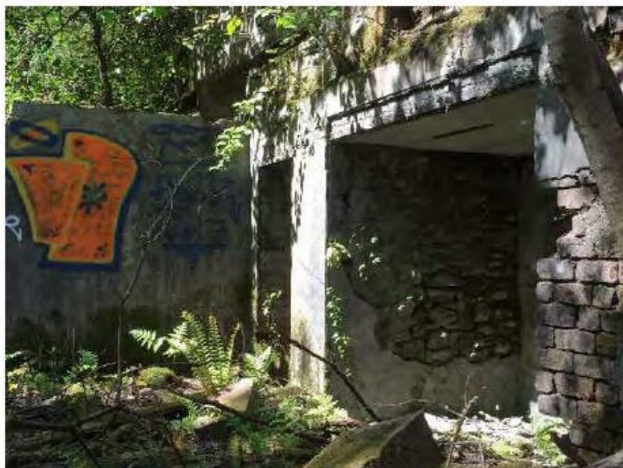
Photograph 17 – Internal views of south block
