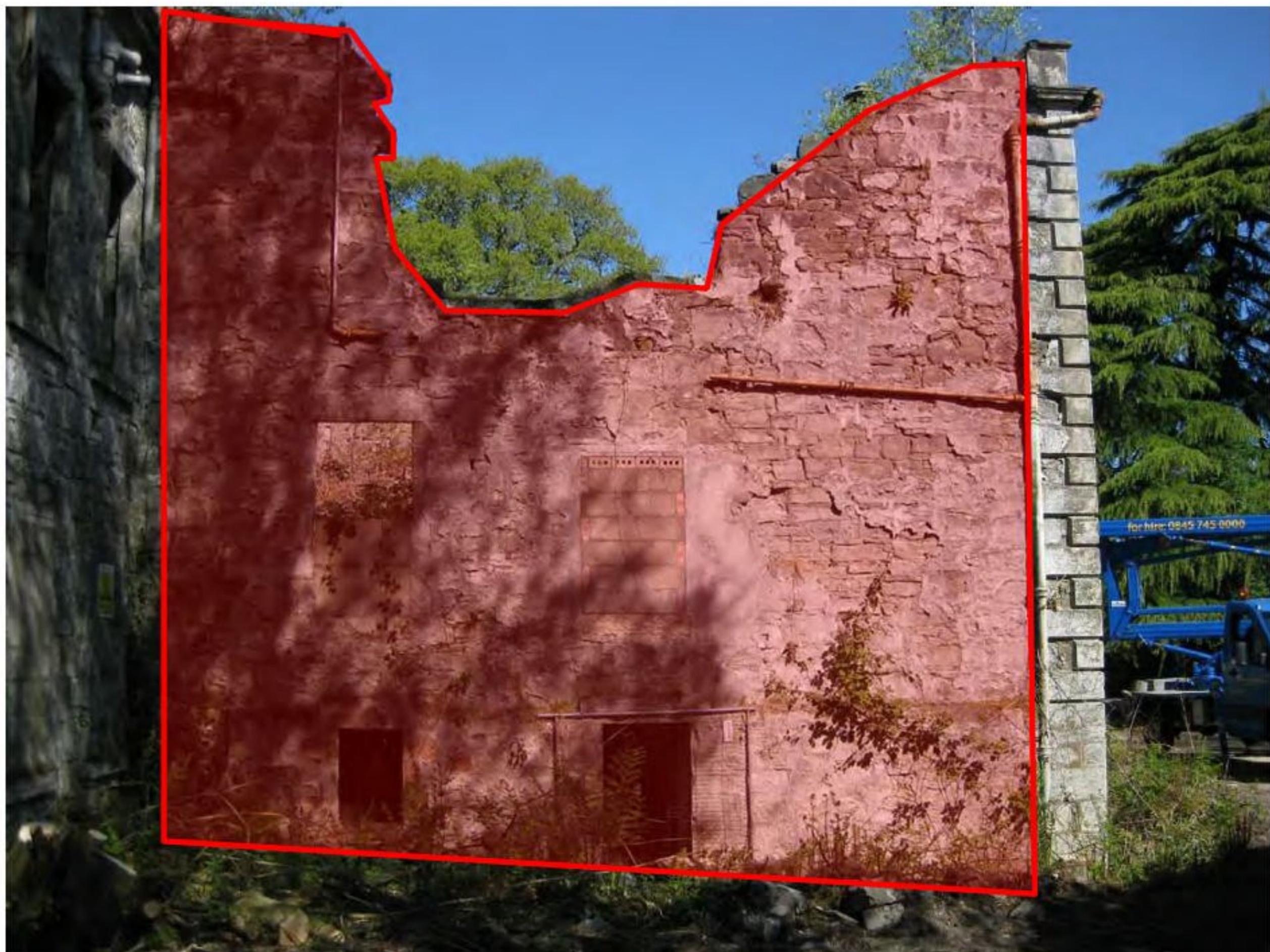
Photograph 3 - South East Elevation Down takings for safety shown in red.
