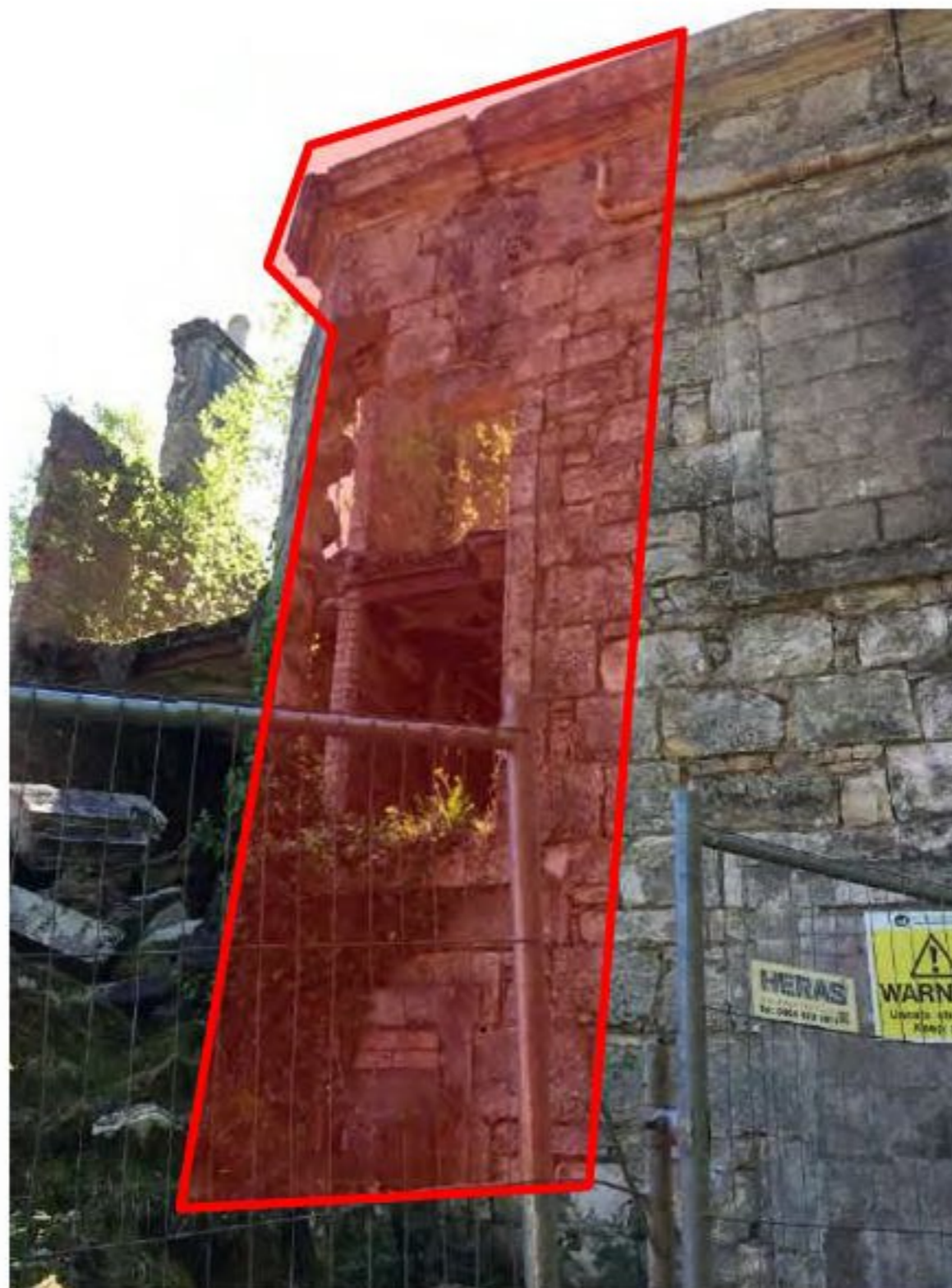
Photograph 8 – North (Rear) Elevation – East section Priority down takings highlighted red.
