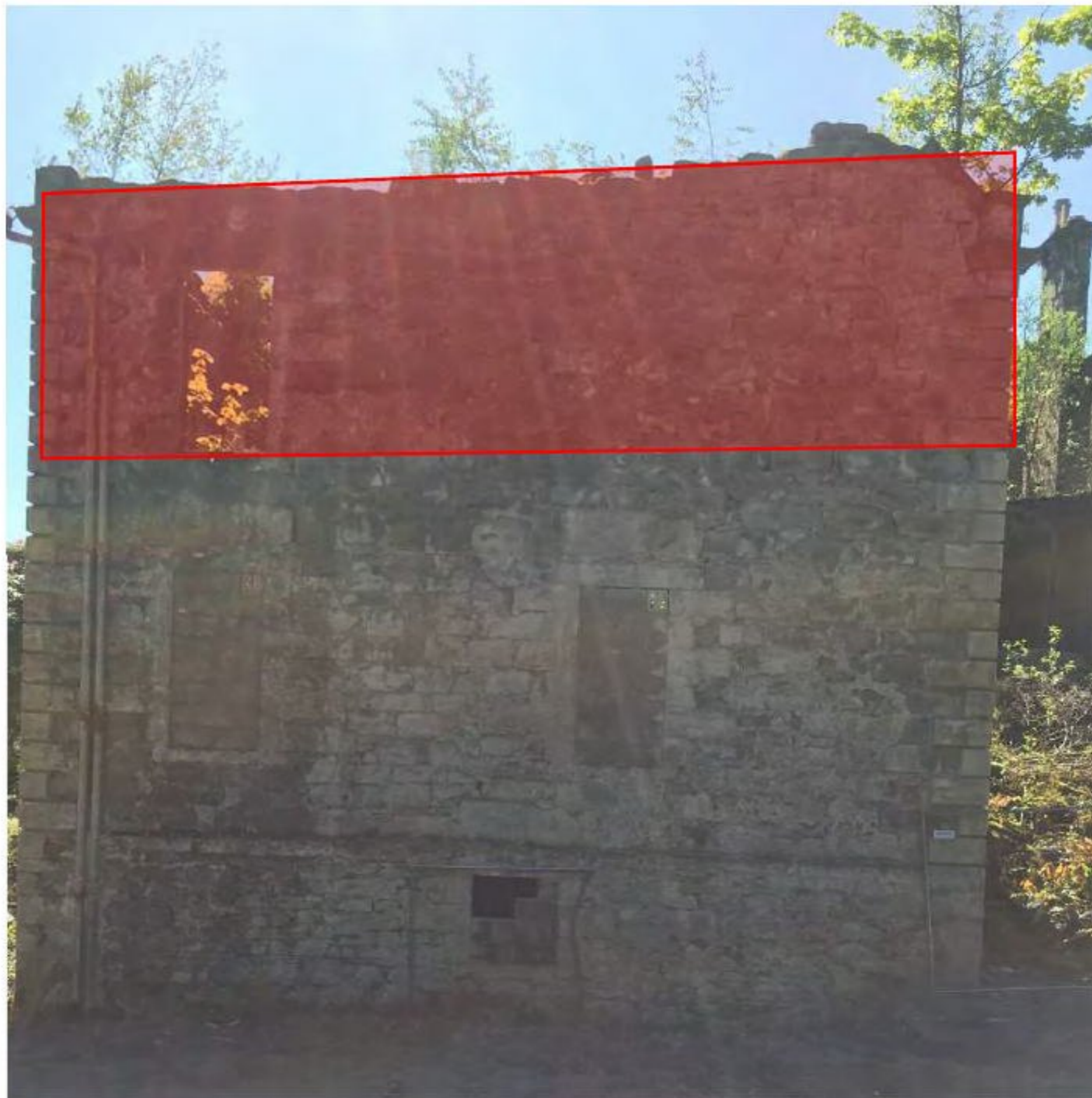
Photograph 11 – North east Elevation Down takings highlighted in red.
