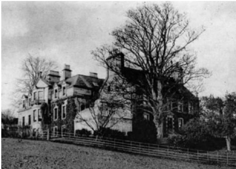
Historic View of Woodbank House showing relationship of original and extended Fascades
