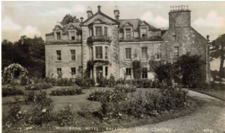
Historic View of Woodbank House from the south east showing manicured garden
