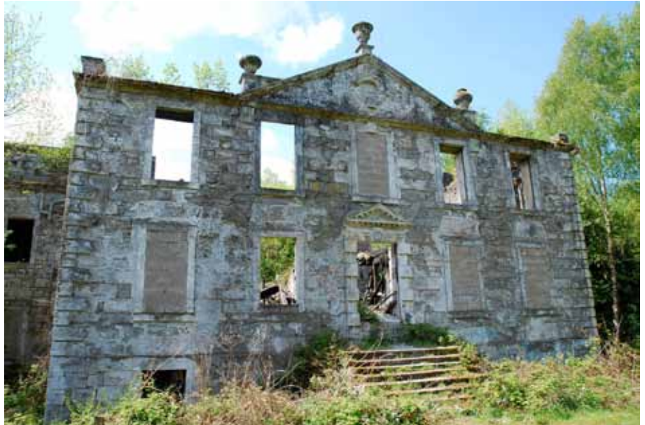
East façade of Woodbank House
