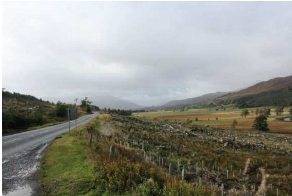
View A: Looking south-west along Glen Dochart
