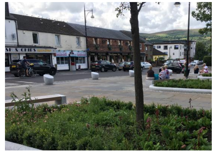
Village square completed works
