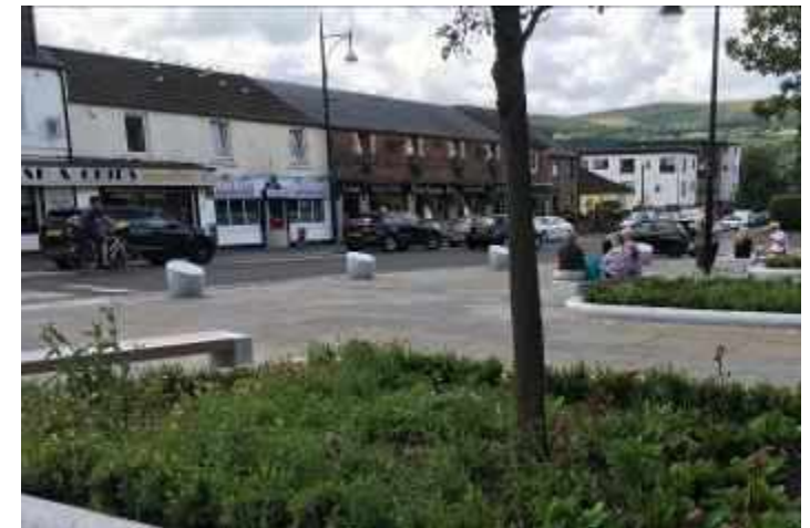
Village square completed works
