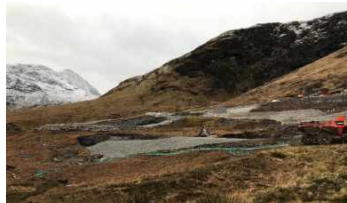
Cononish Glen – Gold Mine Under Construction Jan 2020
