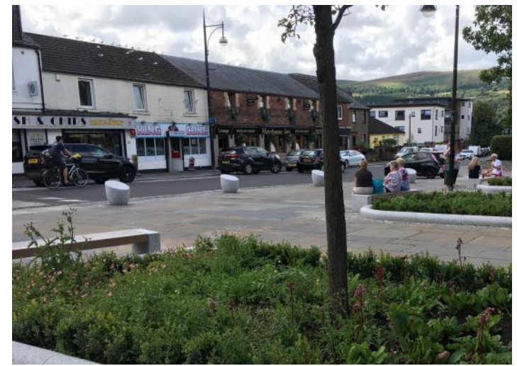
Village square completed works
