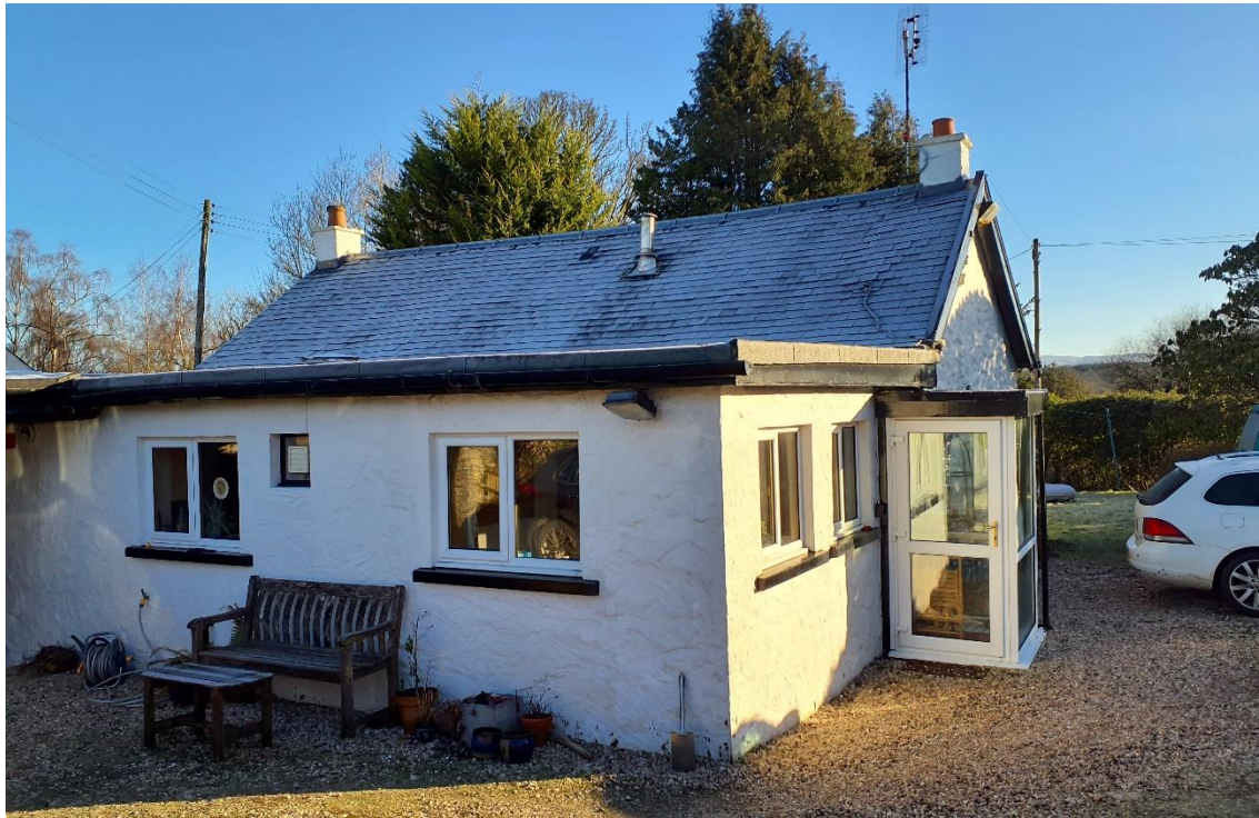
Figure 6: Photo of Aber Cottage showing the later flat-roofed extensions and adjoining stone garage (far left).
