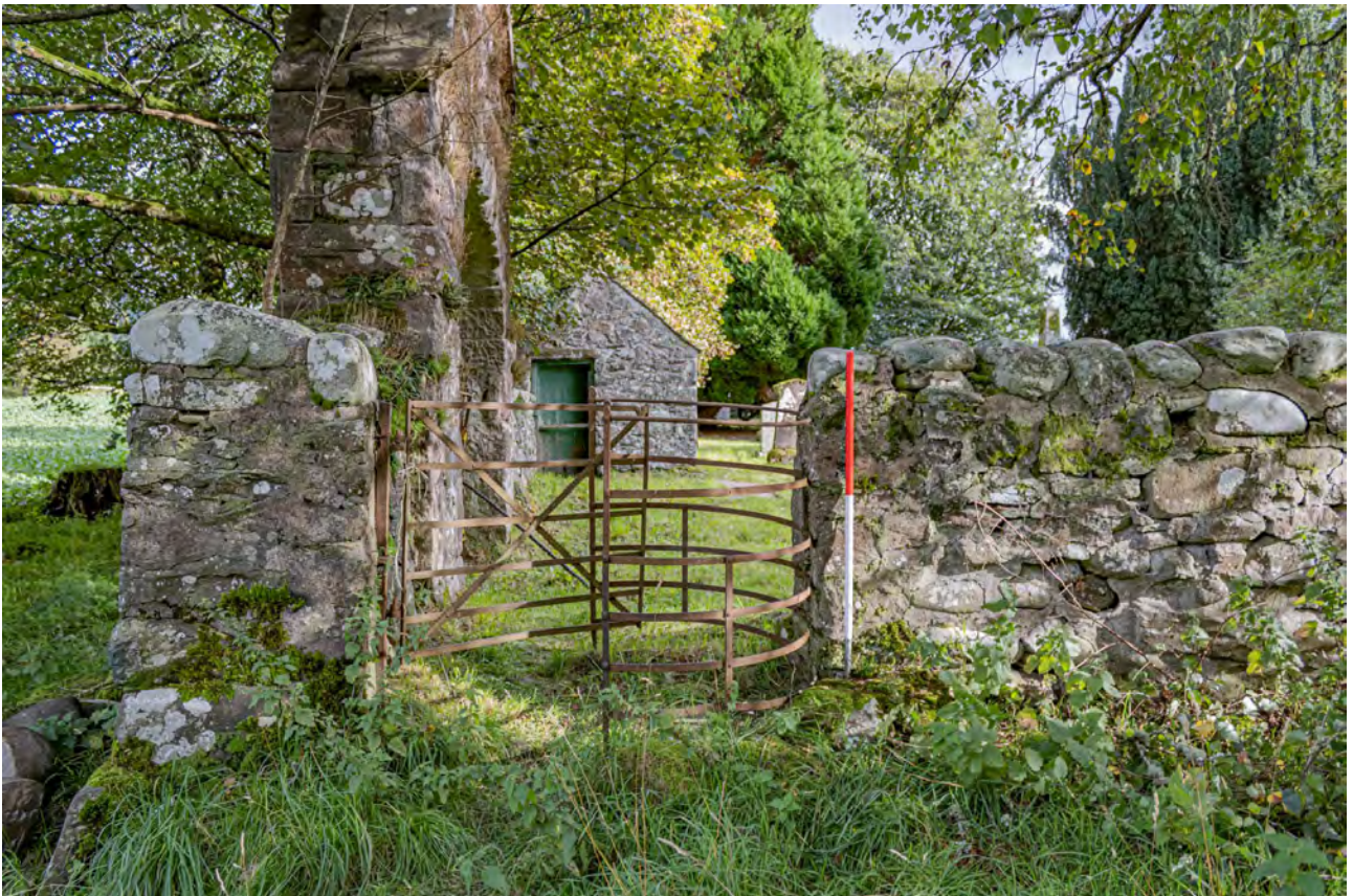
Plate KG7: Kilmahog Graveyard, west boundary wall, detail of the iron kissing gate from the west
