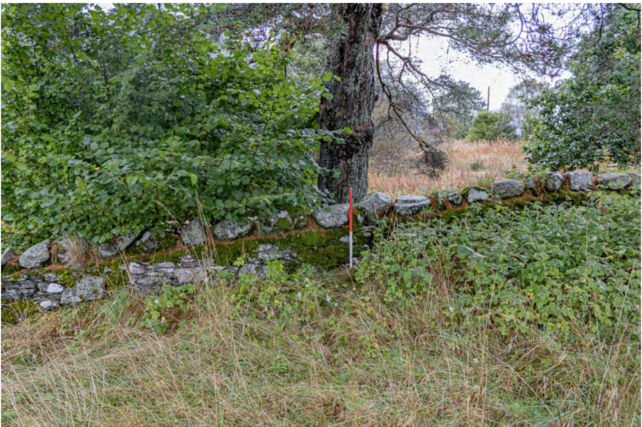
Plate SB2: Saint Bride's Chapel, north enclosure wall, general view from the south
