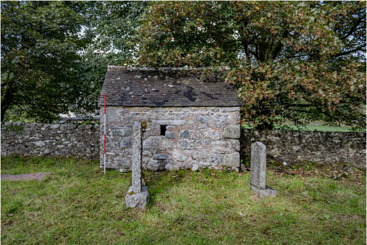
Plate KG10: Kilmahog Graveyard, Morthouse south elevation, general from the west
