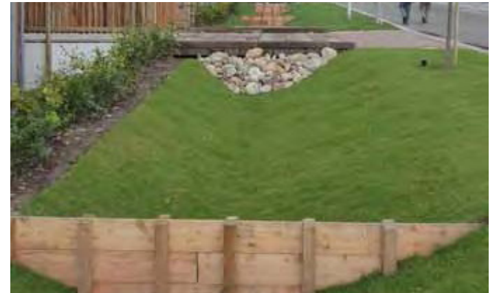
Example of a successful swale, with building entrance bridges over
