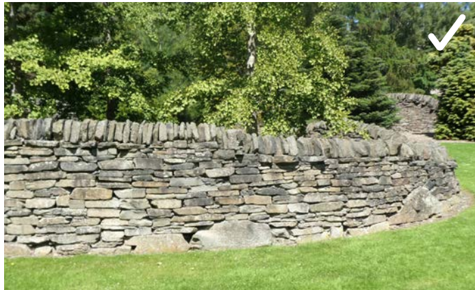
Good example of stone boundary wall
