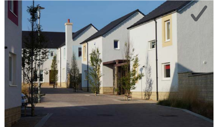
Good example of building frontages unencumbered by parking (c. Proctor and Matthews)
