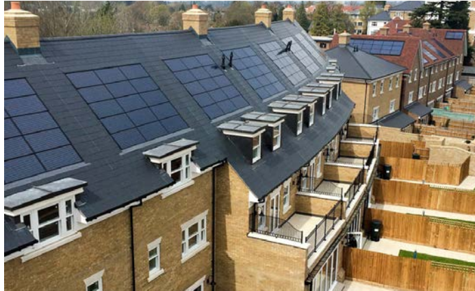
Example of integrated in-roof solar panels
