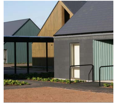
Example of stained timber cladding (c. OCA)
