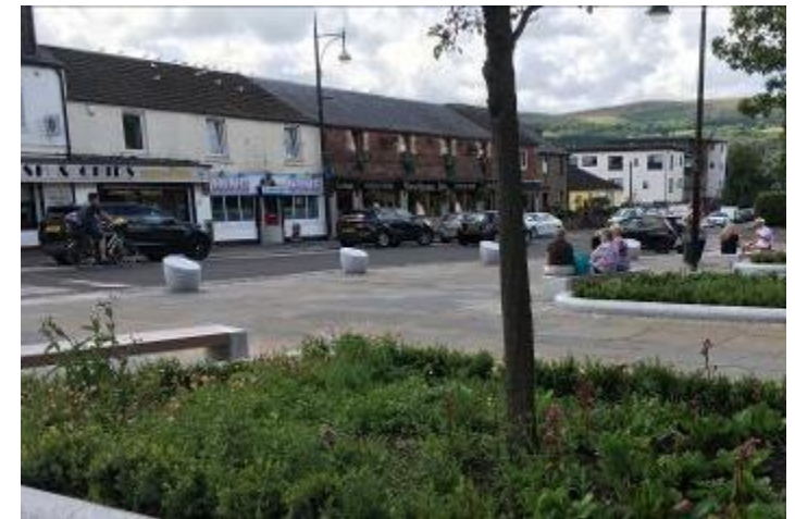
Village square completed works
