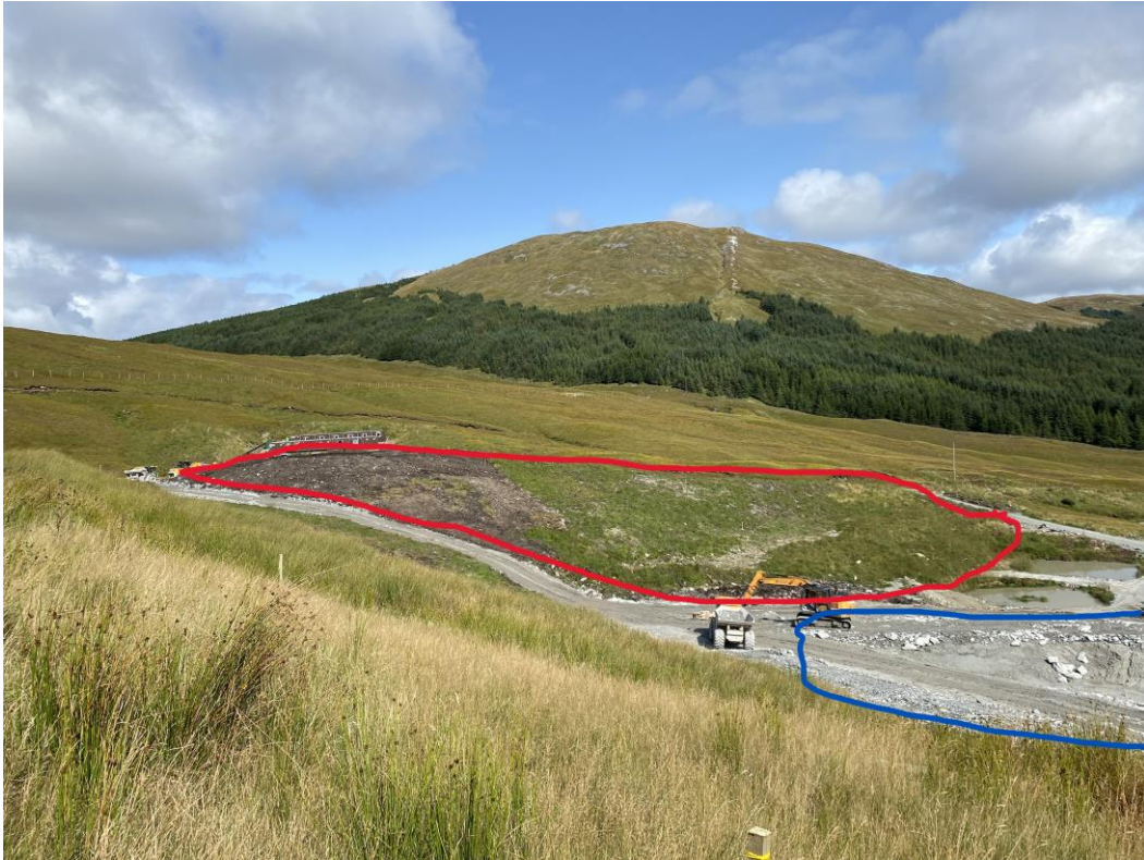
Image 1: View of stack 1 (red) and stack 2 (blue) (August 2023)
