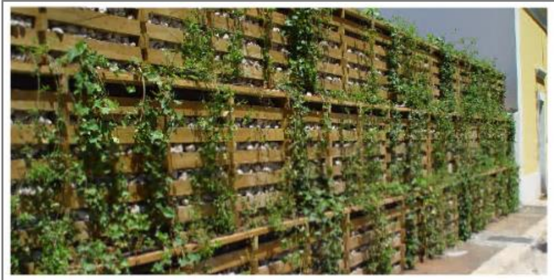
Figure 15: Proposed Crib Walling – Typical Appearance
