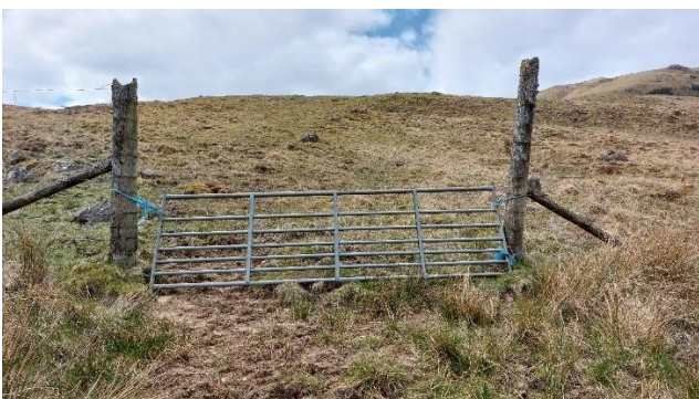
Before: broken gate and deer fence
