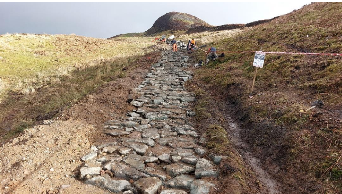
Stone pitching, path section 4 above Bealach Ard
