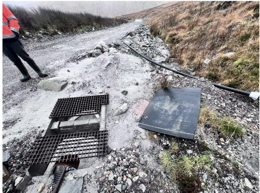
Oil interceptors have been cleared and are functions
