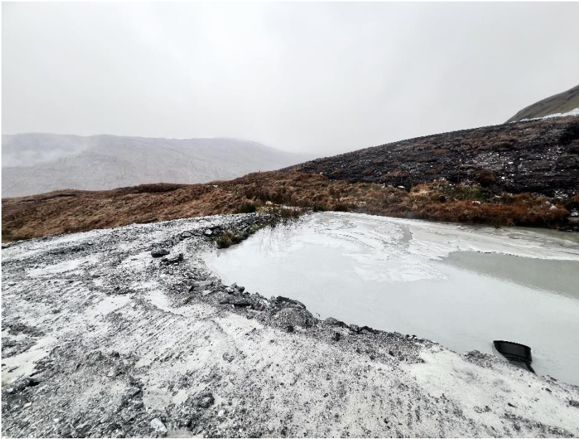
Seepage channel entering the existing settlement lagoons, the build up of sediment requires clearing as part of maintenance works to maintain settlement capacity.
