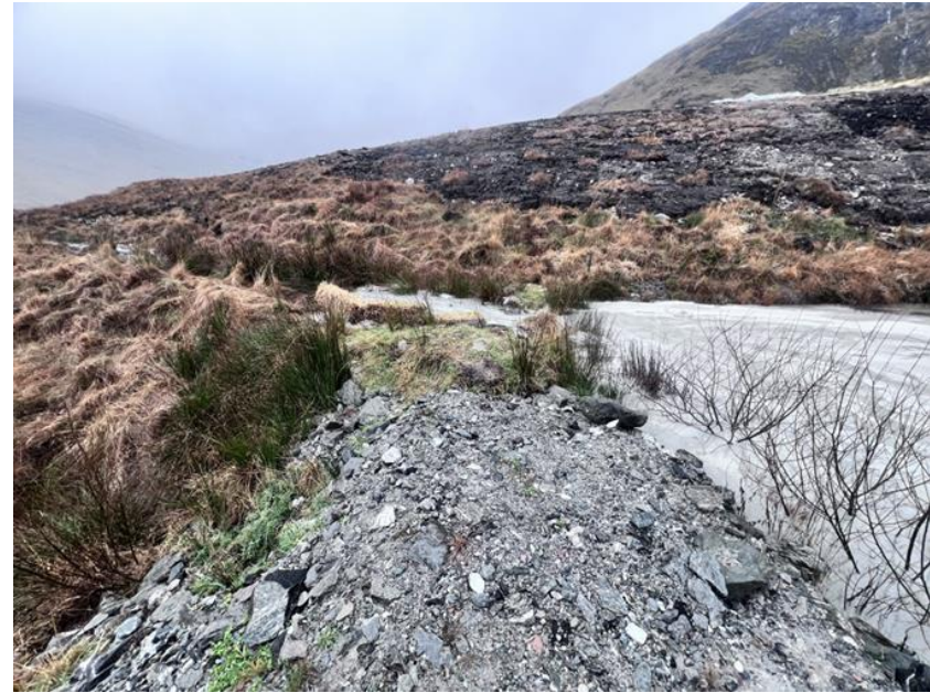
Seepage channel entering the existing settlement lagoons, the build up of sediment requires clearing as part of maintenance works to maintain settlement capacity.
