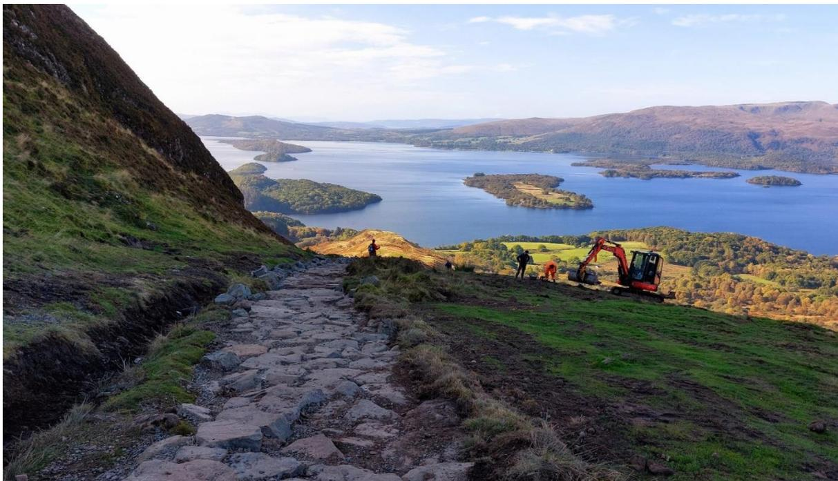
Preparatory work started on the summit path in October and the team are currently breaking up sections of bedrock outcrops prior to the pitching being laid. Unfortunately, due to a combination of half term leave, vehicle breakdowns and illness, 2 weeks were lost in mid-October, and it is now anticipated that the primary path work will be complete in mid-January rather than the end of the calendar year.
