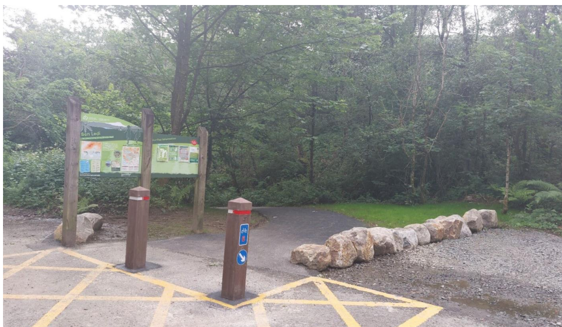
Image: a photo of the improved entrance to NCN7 at the Ben Ledi carpark showing a smooth tarred surface with wooden posts, yellow floor markings and boulders separating the path from the carpark.
