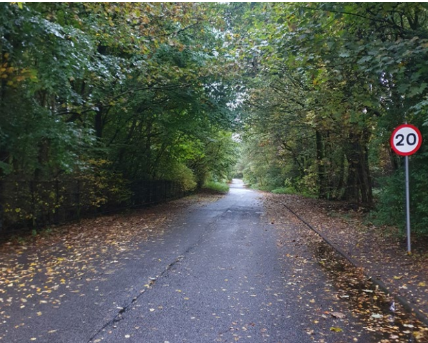
Pier Road: Existing Condition
