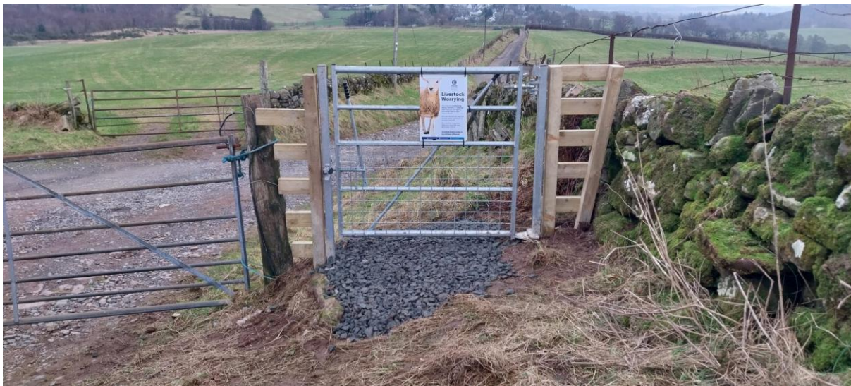
New handgate installed on the route in January 2026.
