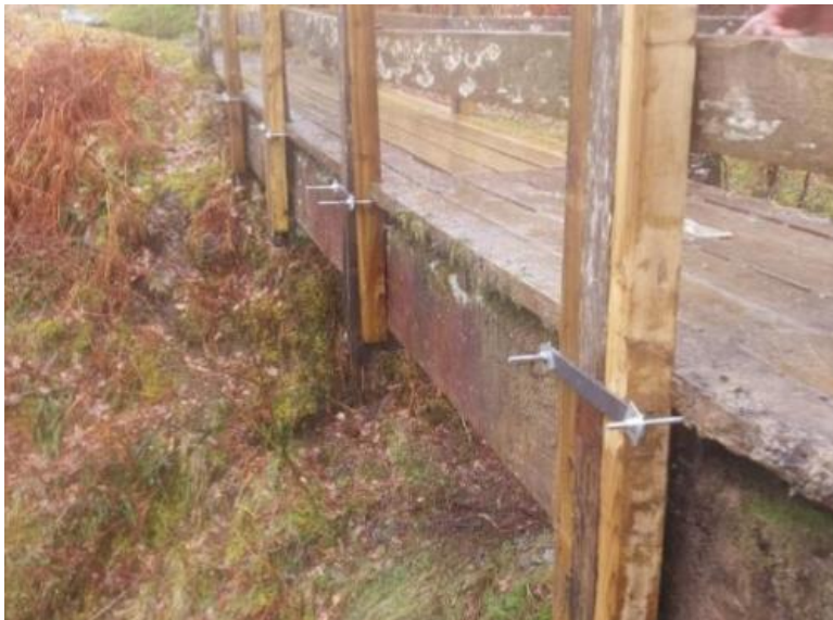
Falls of Falloch - Handrail bracing
