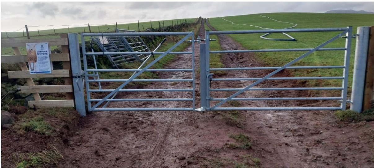
New 2-part gate installed January 2026.
