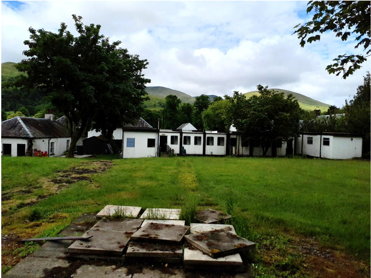
Figure 7 Portacabins sited within the walled garden
