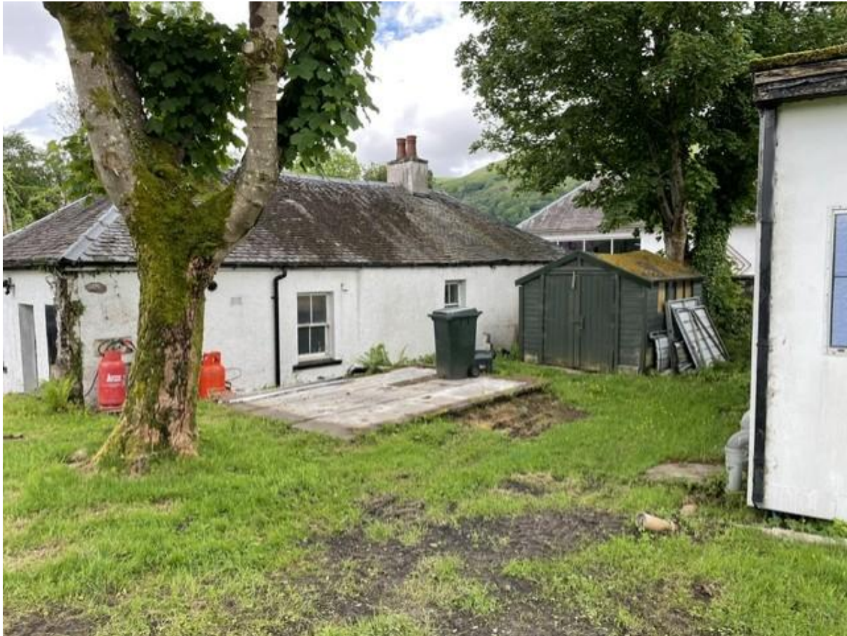
Figure 9 Rear of Manse Cottage – portacabin, shed and trees
