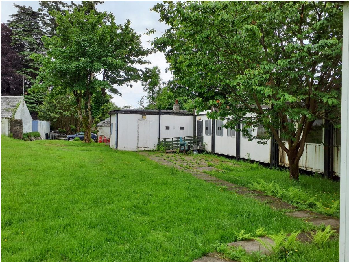
Figure 8 Portacabins – view from within walled garden looking south
